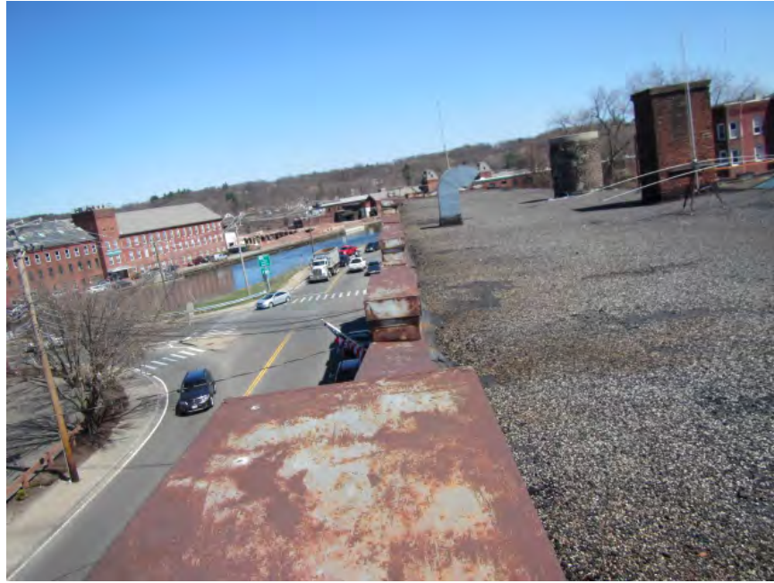
Parapet at front of building
