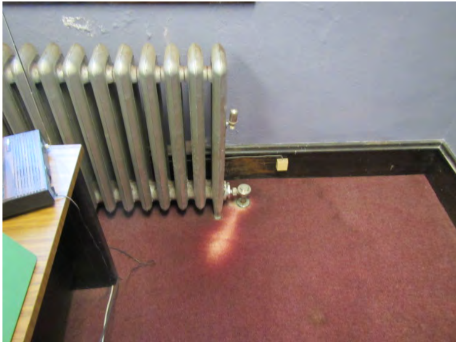
Water-damaged carpet
