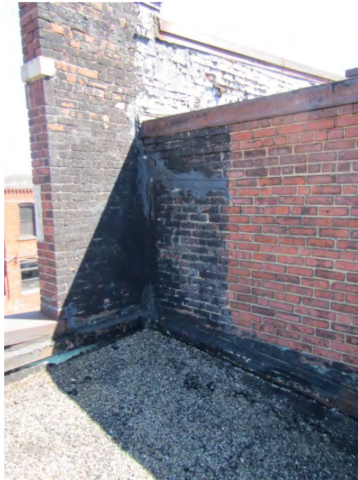
Crack in wall above garage bay
