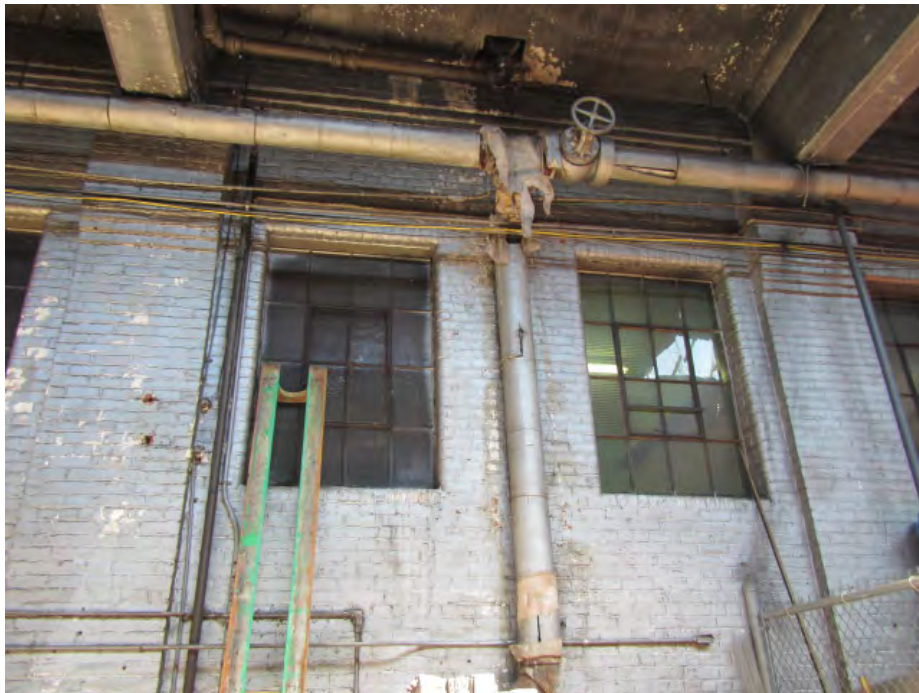
Shared windows between vehicle area and office areas
