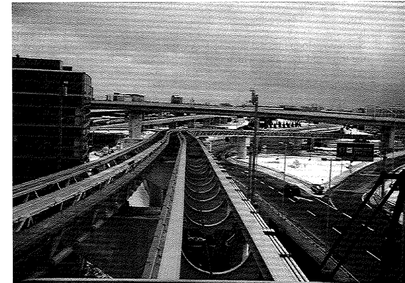
FIGURE 18.11 Double guideway for the APM system at Toronto Pearson International Airport.
