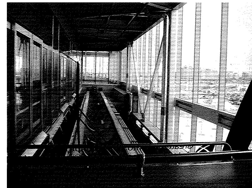
FIGURE 18.15 Maintenance and storage facility at Pearson International Airport in Toronto, Canada.
