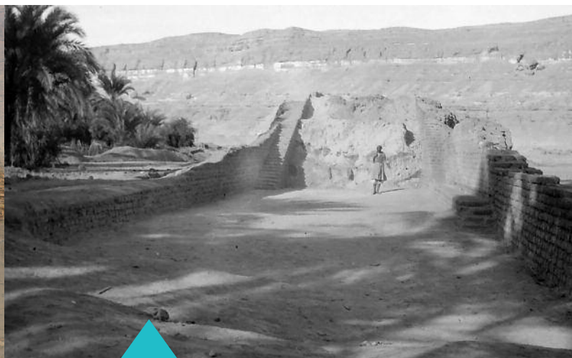
Photograph taken in 1930-31 during the excavation of the double wall. EES Lucy Gura archive photograph 30/31.203.
