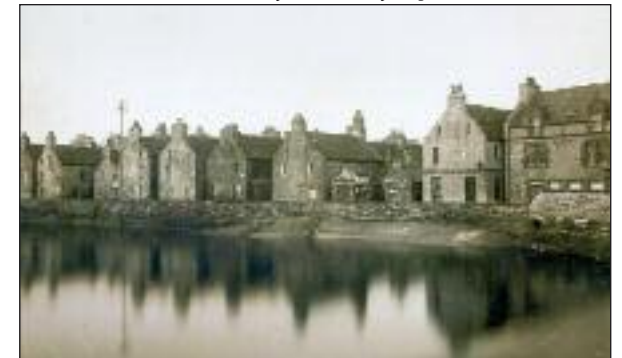
Shore Street before demolition for replacement with BP oil tanks
