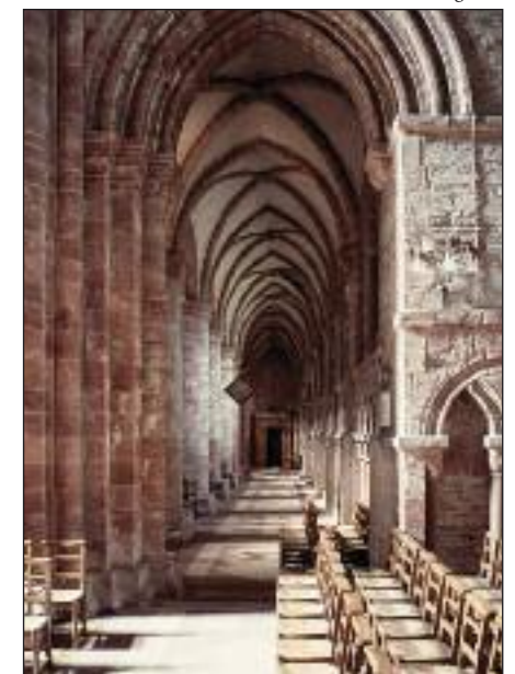
Northwest aisle looking west
