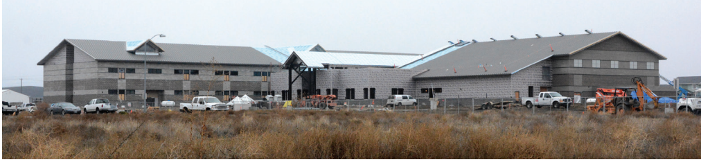
Curie STEM Elementary School is pictured under construction Jan. 28, 2015.
