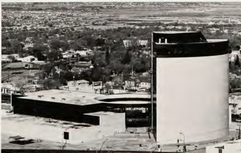
THREE SIDES of the Las Vegas City Hall highrise seem almost entirely of glass. BELOW — A southern view of the complex presently being completed by Webb builders reveals a solid convex travertine marble exterior, an architectural acknowledgement of the abundance and power of the Southwest sun.
