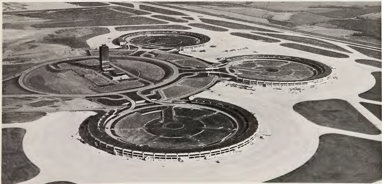
AIR VIEW of Webb construction progress on three terminals at Kansas City (Missouri) International reveals a circular con-
