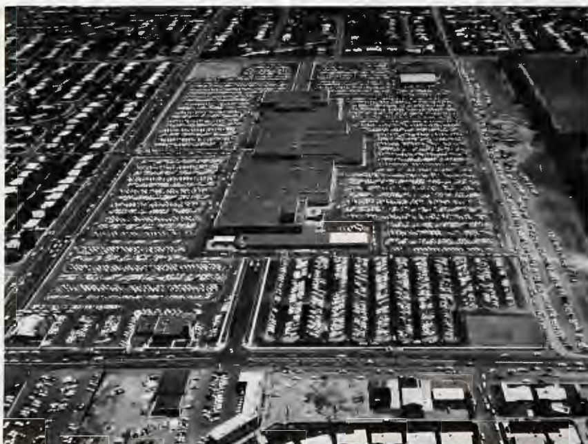
WEBB CORPORATION believes it can claim several "firsts" in Arizona parking facilities, including Chris-Town, the first shopping center with parking for more than 5,000 cars. Aerial photo is of 1961 opening day for Chris-Town, which Webb owned and operated for three years.
