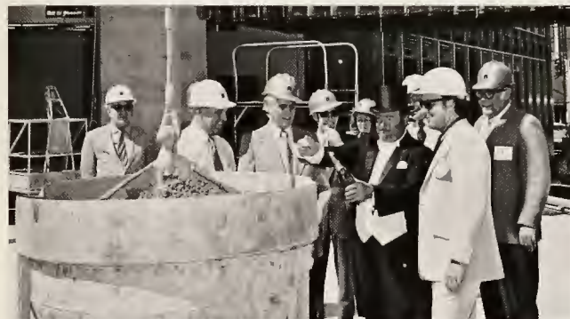
ARRIVAL of last bucket was timed to appearance of Will Hughes, labor foreman, who uncorked the bottle to mix contents with wet concrete.
