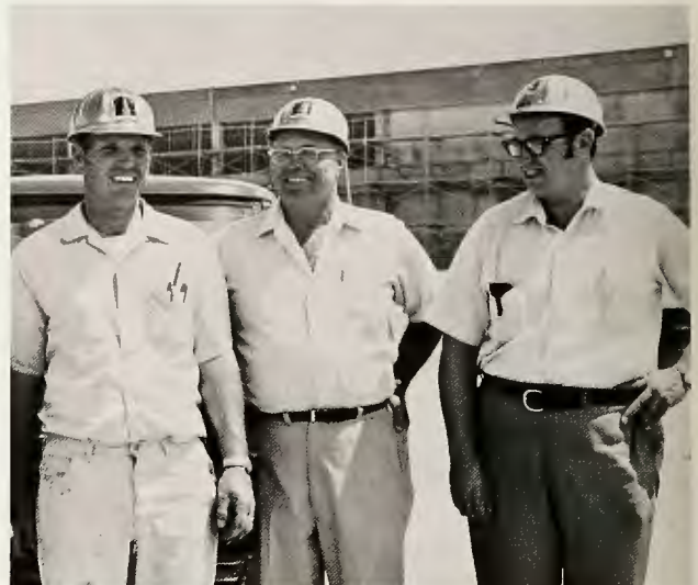
CLARK County's (Nevada) newest high school was about 60 per cent complete and on schedule in early June when this photo was taken. Construction is guided by Webb crew, from left: Guy Thomas, assistant superintendent, Bob Gray, superintendent and Pat Haisch, engineer.
