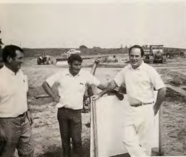
GRESS on Wabeek course is surveyed by Pete Dye, right; his er and associate, Andy, left, and Max Robertson, construction ntendent.
