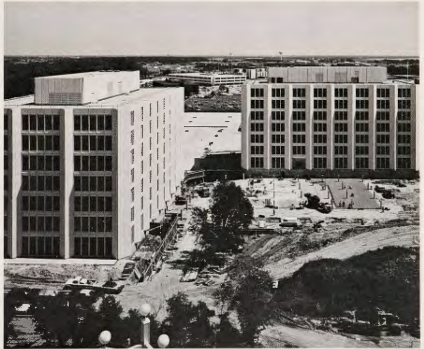
TWIN OFFICE buildings and garage in Oak Brook, Ill. for Arthur Rubloff & Company, near completion under direction of Don Kosman, superintendent; Walter Bombard, operations manager; Carolyn Moore, engineer and Charlie Brown, office manager.
