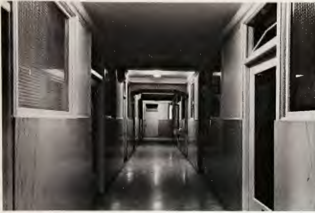
BEFORE — Typical office hall, era 1920s.
