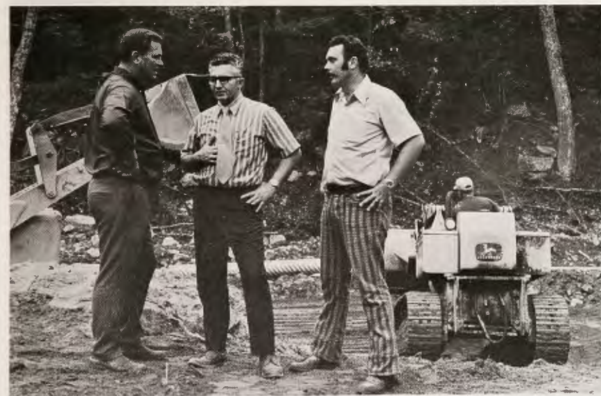
TOM RILEY, right, manager of project operations at Massanutten, is an excellent skier who is involved in day-to-day construction of the project's first five slopes. With Riley, at a Massanutten road-building site, is Len LaSala, center, general manager and Bill Raycraft, chief of operations.
