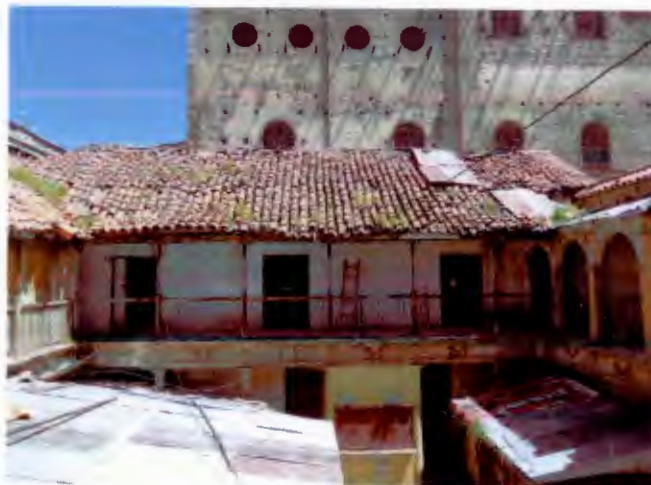
Patio Interior principal
