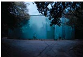
Mira Monte Reservoir
