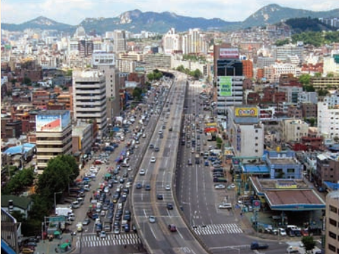
a. Elevated freeway
