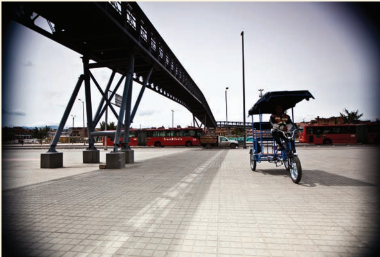
Figure 4.4 Flyover in Bogota's TransMilenio bus rapid transit system
