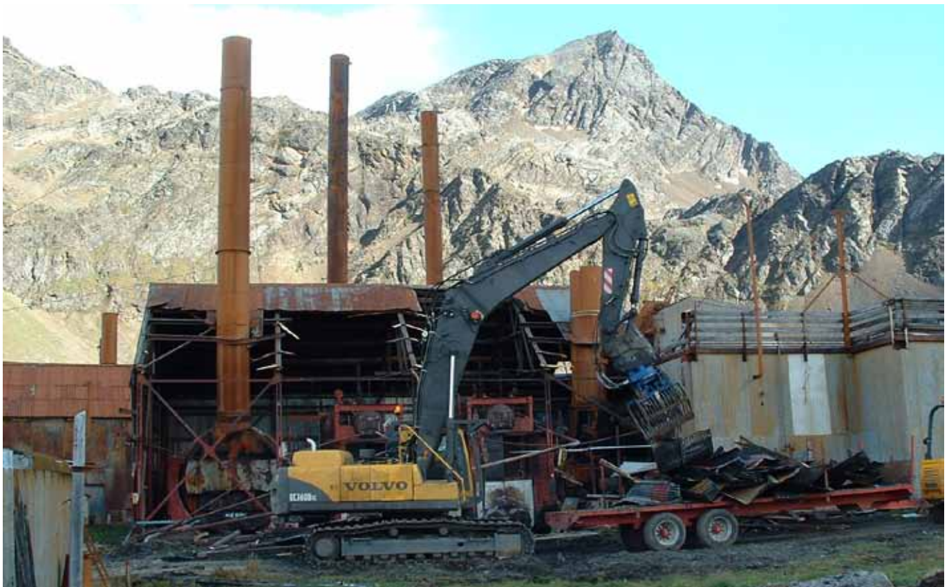
Demolition of the Boiler House in 2003
