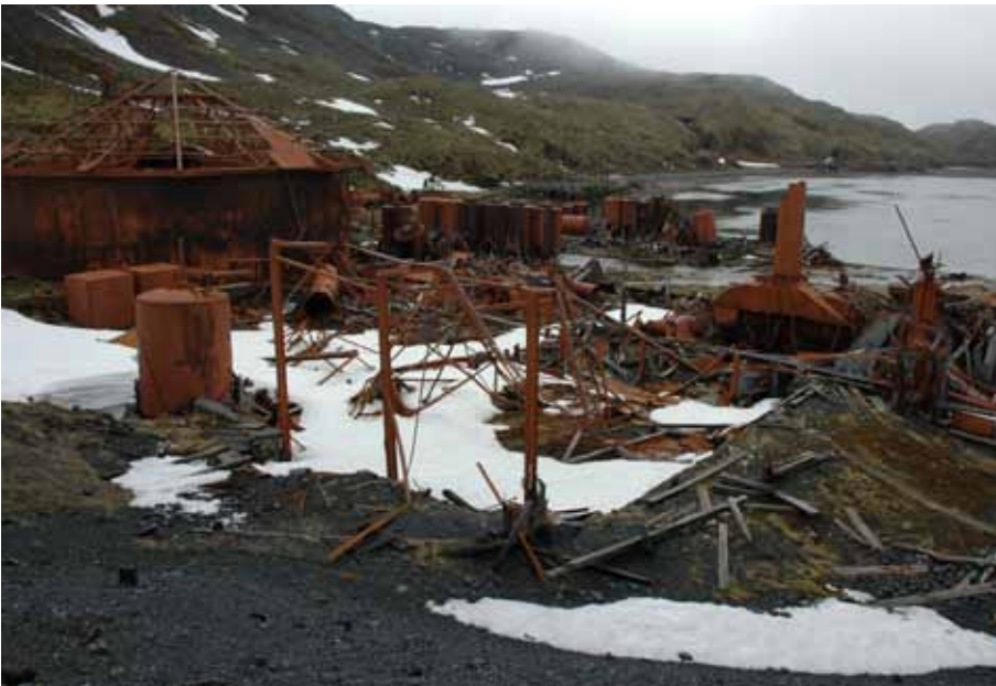
The Boiler House looking northeast at Prince Olav Harbour
