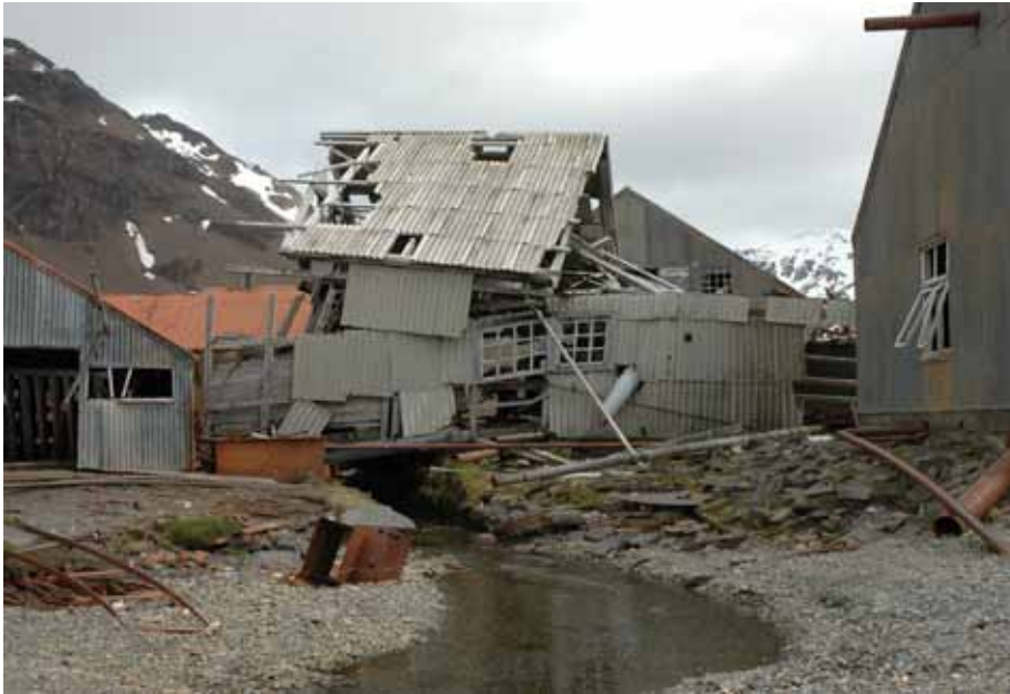
The separator and Glue Water Plant building (No. 5) at Husvik
