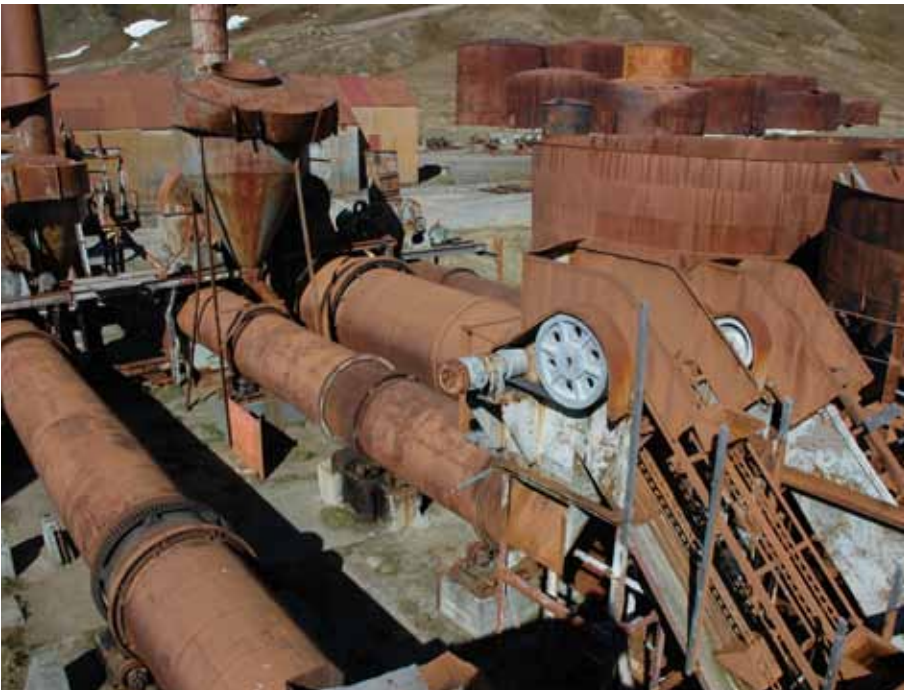
The machinery inside the Guano Plant now out in the open in 2010
