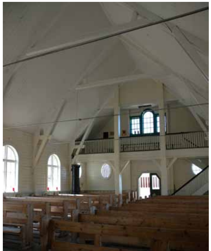
The church today looking east. The thickening of the support posts can be seen.
