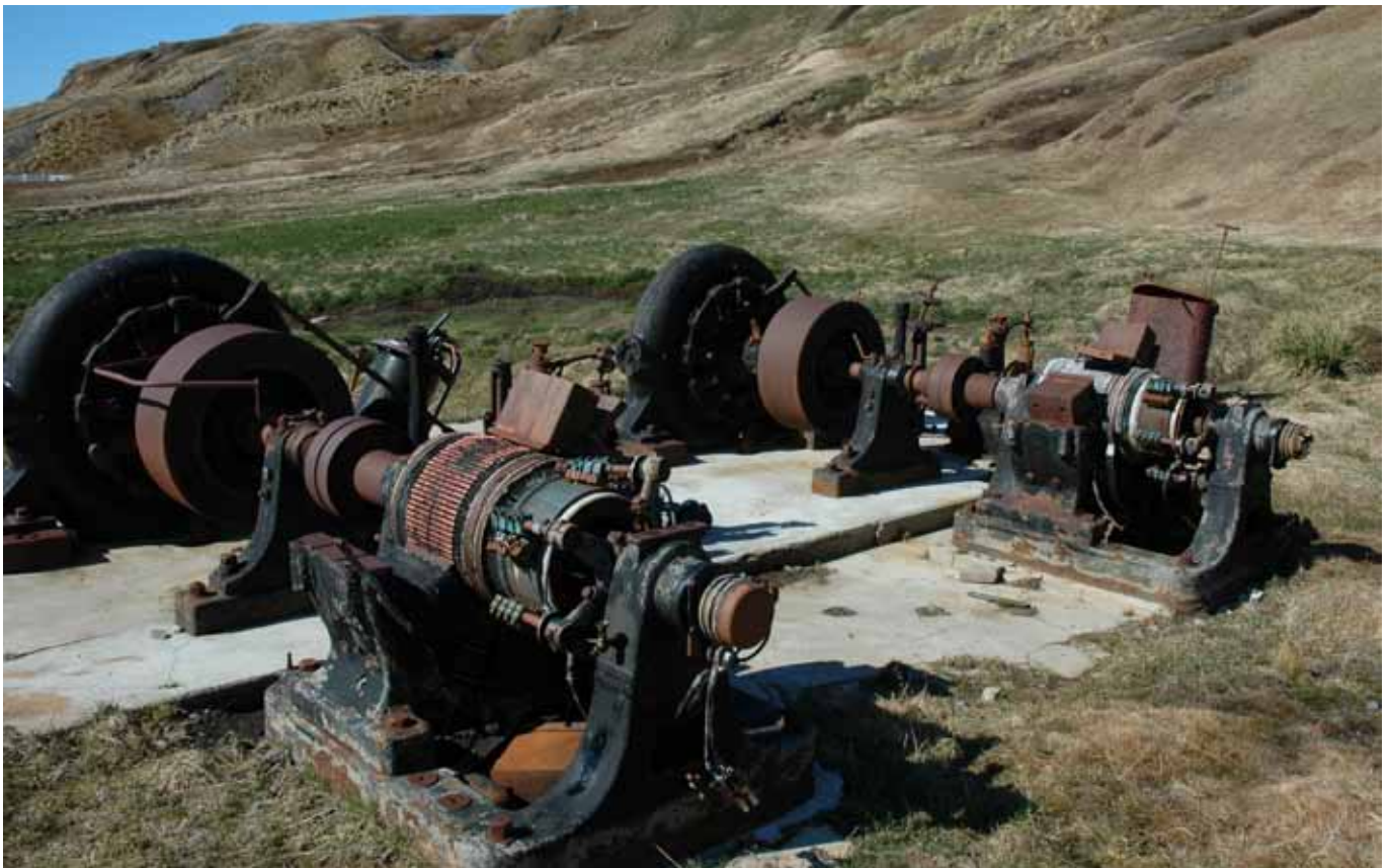
Equipment such as the hydro-electric turbines and generators will need conservation and maintenance if they are to survive
