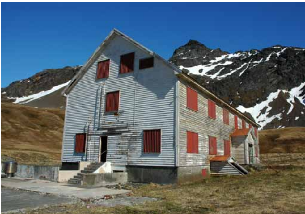
Nybrakka looking westwards with the remains of the earlier mess building in the foreground
