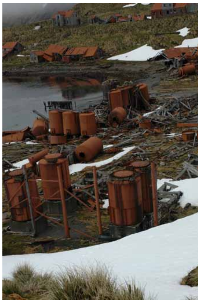
General view over Prince Olav Harbour looking south
