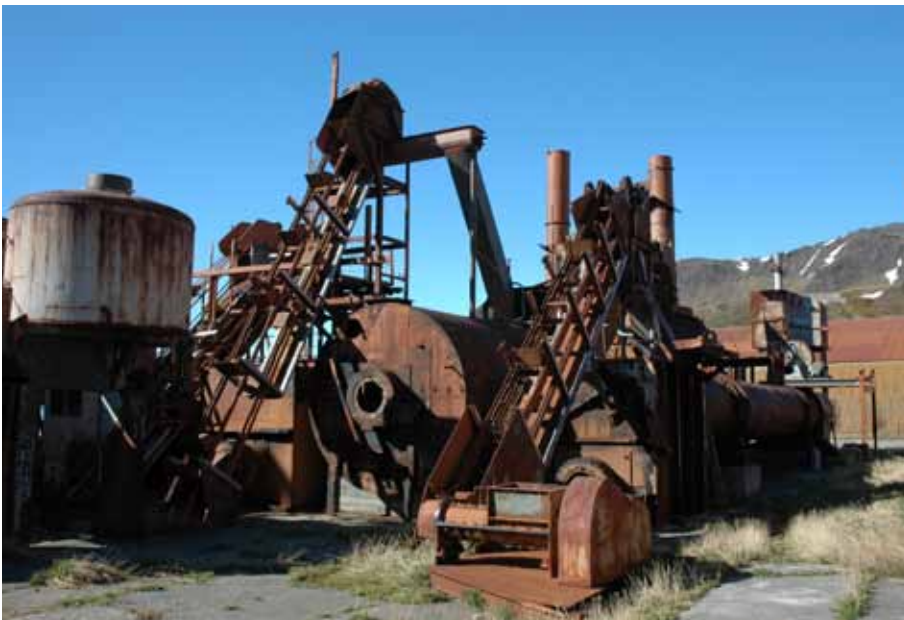
Conveyor equipment for the Guano Plant at Grytviken. There is a large amount of similar equipment at all the sites.
