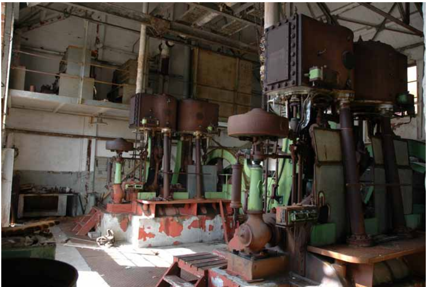
Steam engine and dynamo sets in the Power Station building at Stromness
