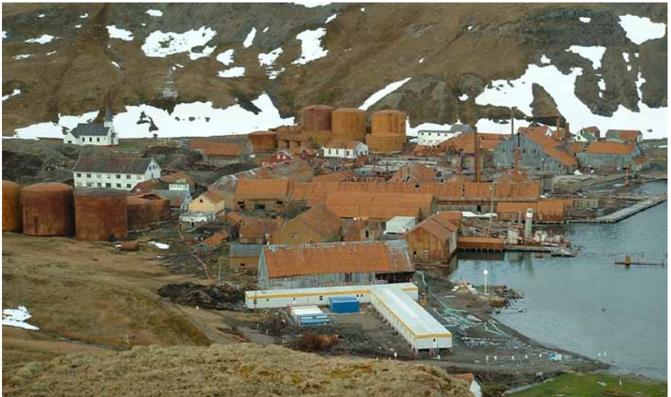
View over Grytviken (looking north) in 2003. Some demolition has already taken place (the cold store in the foreground for example).
