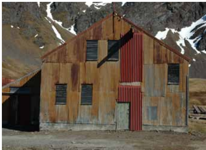
The use of modern wrongly profiled sheet to repair the Main Store east wall
