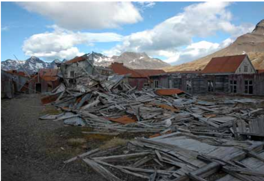
The remnants of the Cinema and Library (No. 24) at Husvik
