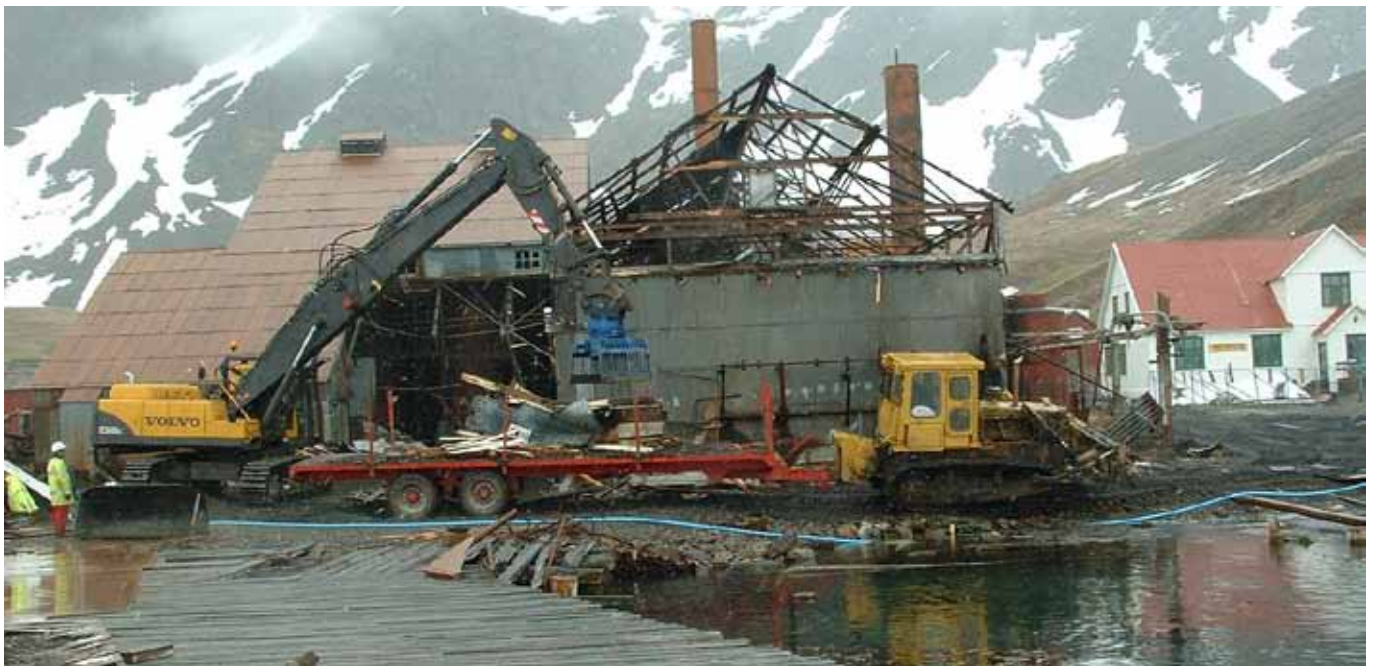
The demolition of the Blubber Cookery in progress in 2003
