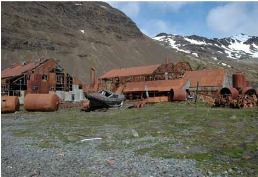
A view across the Flensing Platform with the Boiler House in the centre and the Old Blubber Cookery to the left at Stromness
