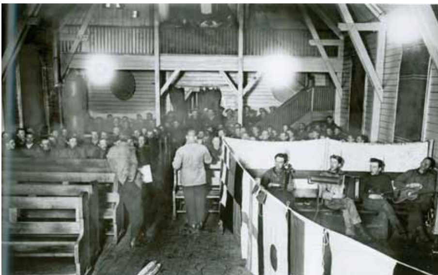
The slenderness of the posts supporting the balcony and the tower are evident in this photograph of the 1920s. (© Grytviken Seen Through A Camera Lens, Institut Minos)
