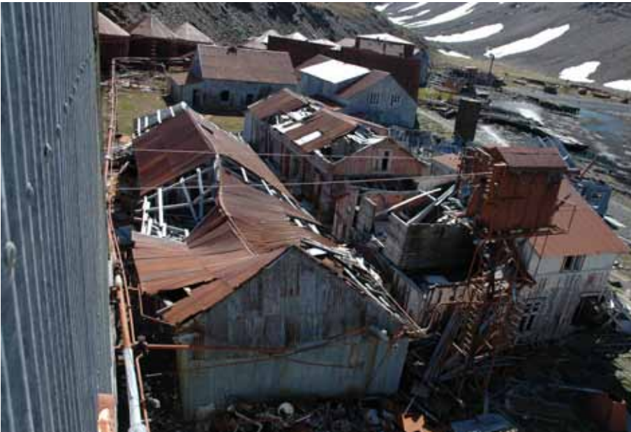
A and C Barracks, Mess and Provision Store buildings (Nos. 53, 63 and 64) seen from the upper window of the Steward's Store
