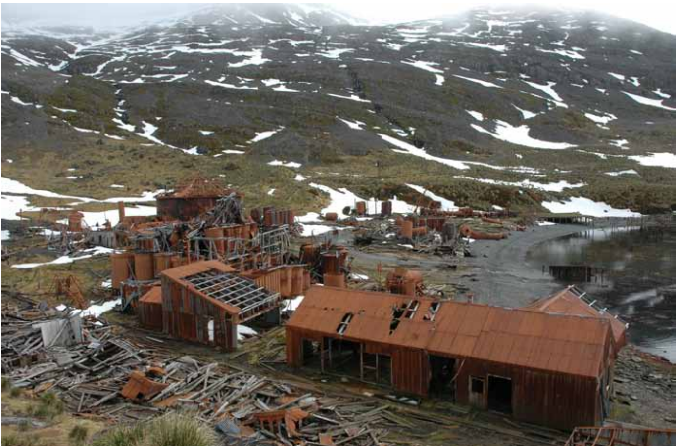
General view looking northwards across Prince Olav Harbour. The relatively intact building in the foreground is No. 14 - The Carpenter and Butcher's Shop.
