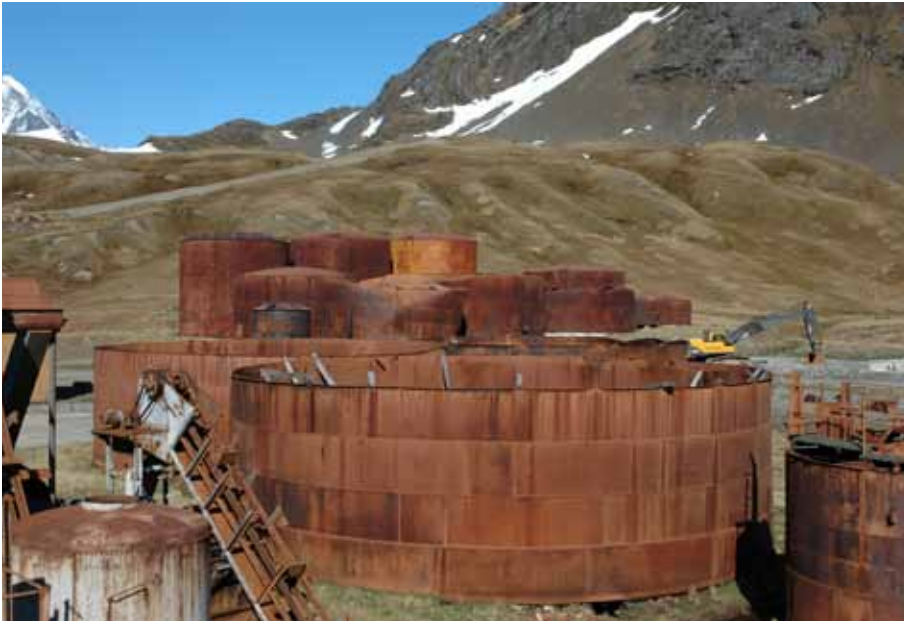
Fuel tanks at Grytviken in 2010. The large tanks in the foreground are the 1920s tanks minus their roofs. The later diesel tanks behind.
