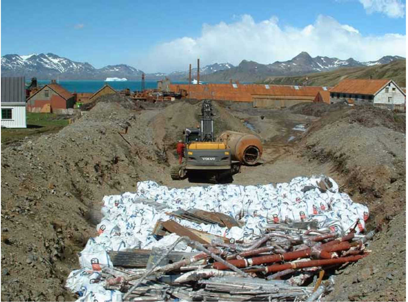
Asbestos being buried at Grytviken in the 2003/04 clean-up campaign
