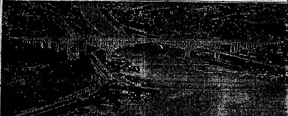
TO BE DEDICATED—National interest centers today on the new George Washington Memorial Bridge, where impressive ceremonies will mark its dedication on the 200th anniversary of George Washington's birth.
