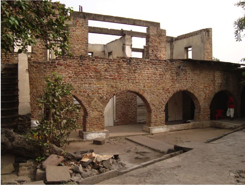
Figure 9. Franklin House, Danish patron(s), c. 1800, stone nog, brick, Jamestown, Accra, Ghana. 2012 (author's photo).
