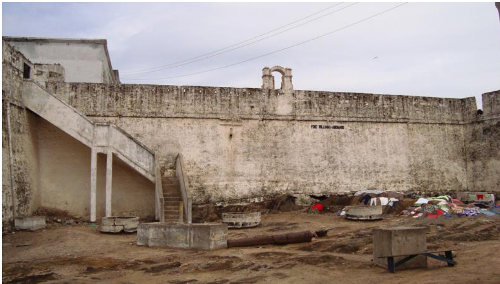
Figure 16. Fort William, North Side, 1760 and 1840s, stone nog (paint added later), Anomabo, Ghana. 2008 (author's photo).
