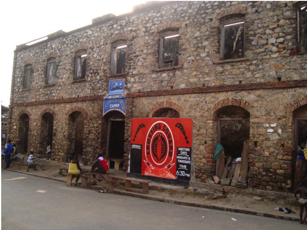
Figure 7. Russell House, façade with club signage. 2011 (author’s photo).
