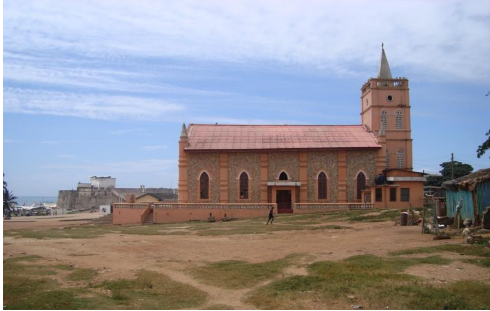
Figure 19. Ebenezer Methodist Church, Revs. James Picot, James Fletcher and John Oboboam Hammond, 1895, stone nog. Renovation 1966-1971, rebuilt main entrance façade, added pilasters and chapel, stone nog, cement and paint. Anomabo, Ghana. 2009 (author's photo).
