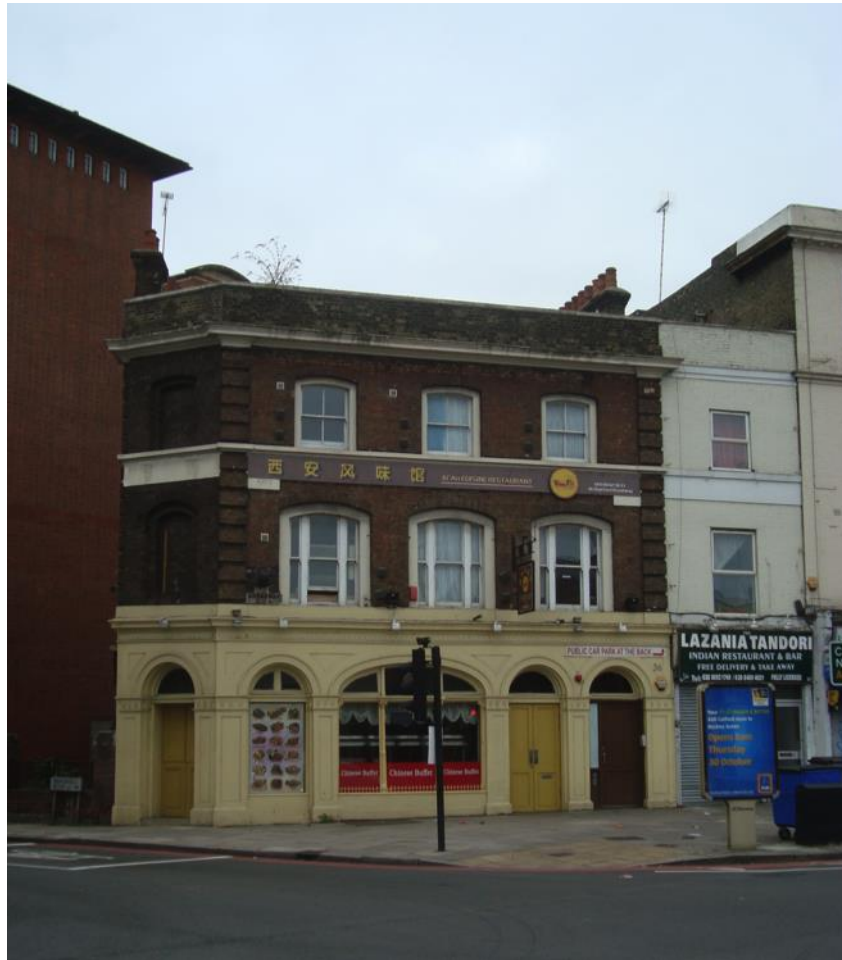
Figure 14. 36 Deptford Road, c. 1860-90, brick, London, England. 2014 (author's photo).
