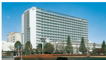
Head Office Technical Center (Toyota City, Aichi Prefecture, Japan)
