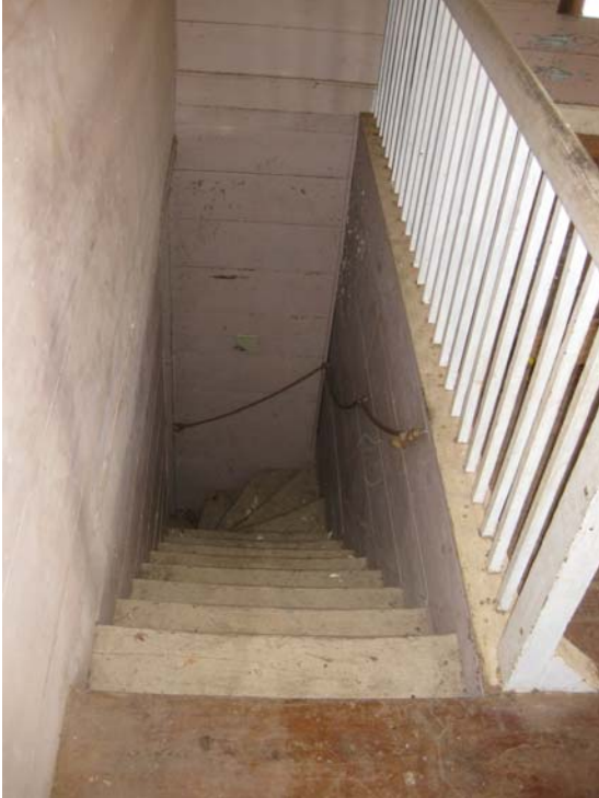
15. Existing Staircase and Railing
