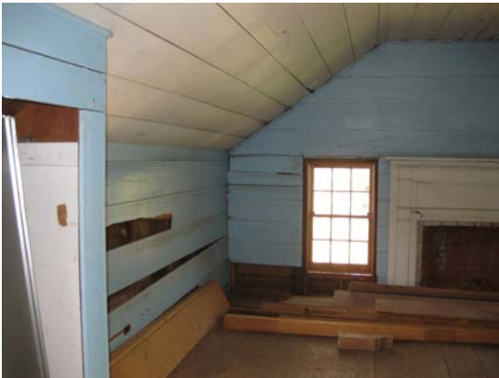
13. Second Floor, West Room
