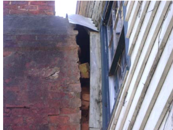
Chimney at exterior, note opening at wall exposing wall cavity
