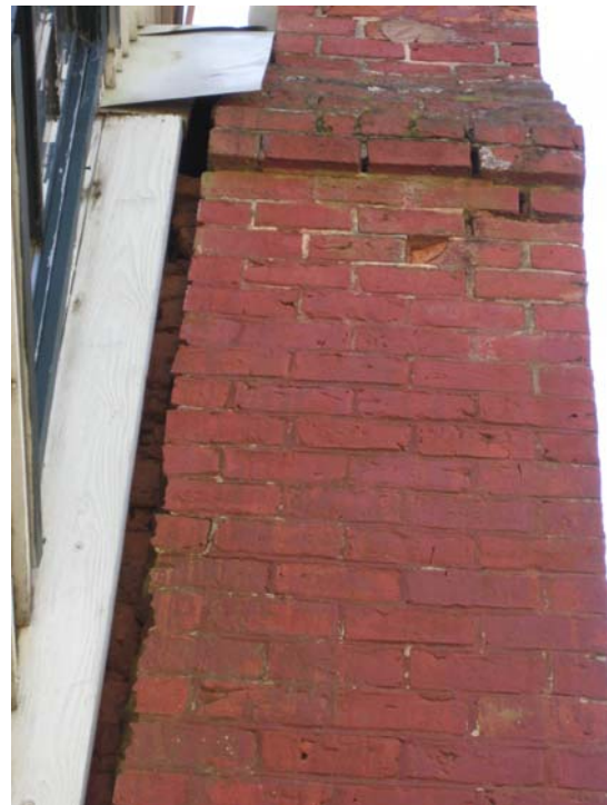
8. Chimney @ West Elevation
