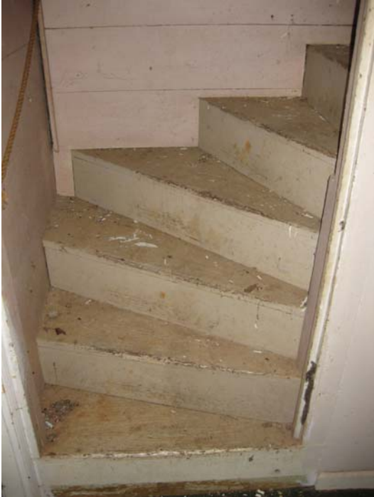
17. First Floor, Existing stair
