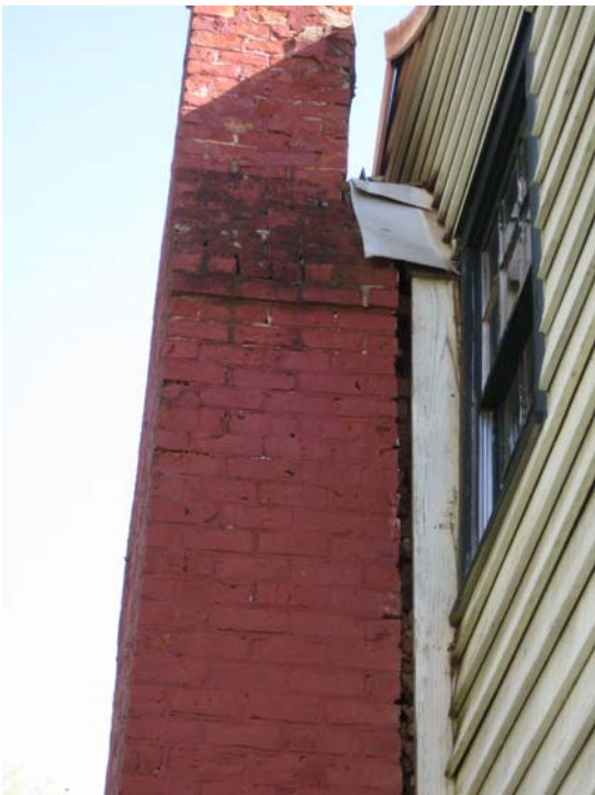
7. Chimney @ West Elevation
