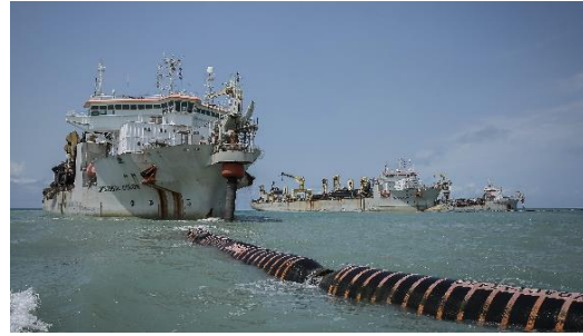
Dredging and reclamation works for Dangote Lekki Refinery (Nigeria)
