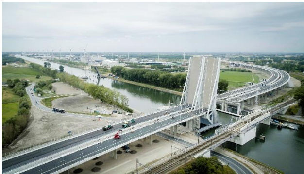
Construction of a new highway A11 (Belgium)
