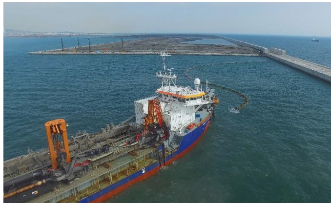
Van Oord completes expansion of Taiwan's largest port
