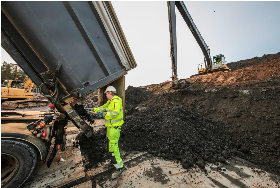
Removal, dewatering and disposal of contaminated sediments in the port of Oskarshamn (Sweden)
