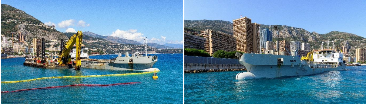
Reclamation works at sea (Monaco)
