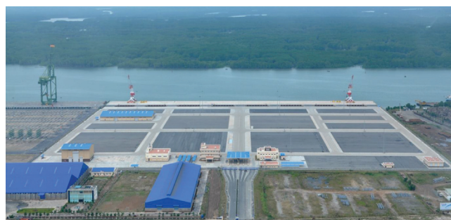
'Hai Phong Port Rehabilitation' ~ 'Hai Phong Port Rehabilitation P2'
