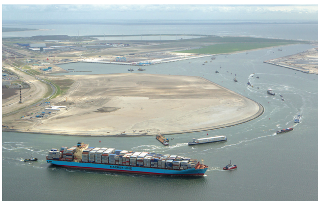
Opening Maasvlakte 2 – Aerial view
