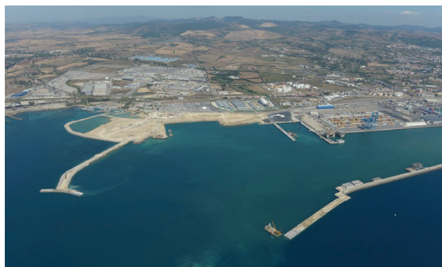
Port of Civitavecchia: Aerial view of the ongoing works
