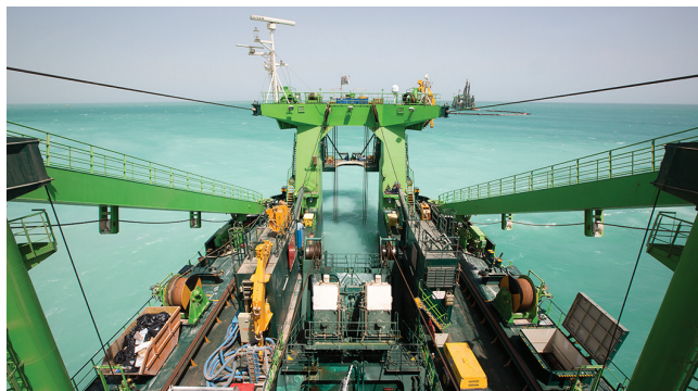
New Port Project Doha
