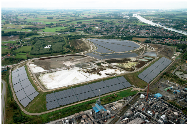
Terranova Solar – Overview
