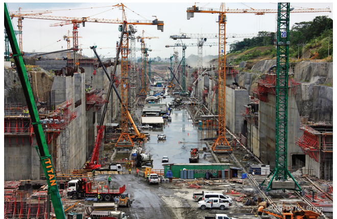
Construction of Third Set of Locks (Panama)
