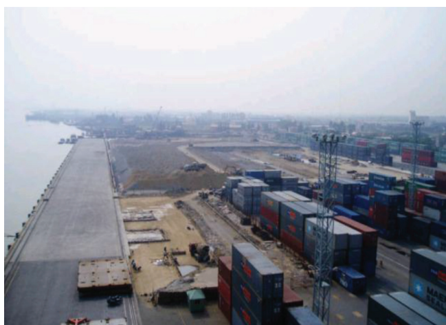
Hai Phong Port Rehabilitation (Phase 2)
