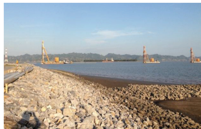
Lach Huyen Port Construction (Package 6)
