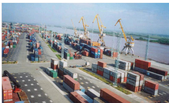
Hai Phong Port Rehabilitation
