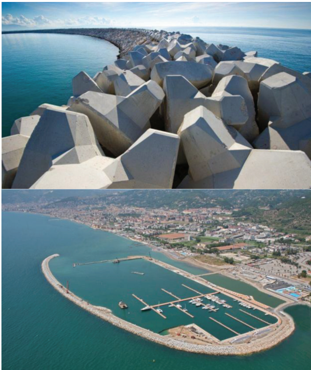
Construction works of Marina di Arechi
