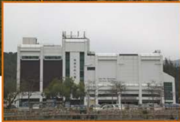
梅窩市政大樓 Mui Wo Municipal Services Building
