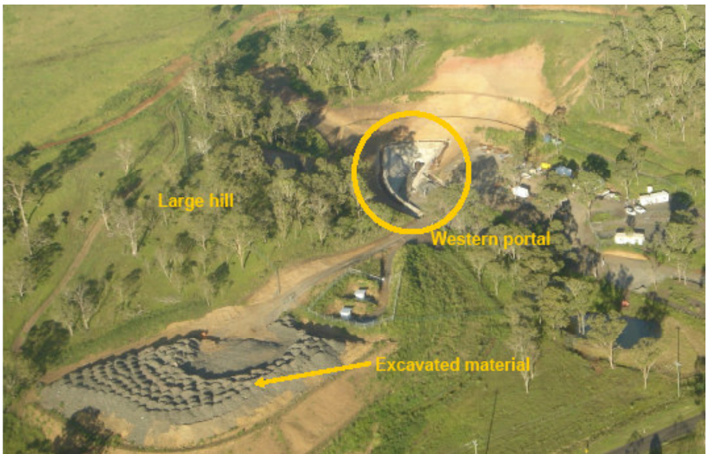
Figure 1. Western portal area showing the location of the completed pilot tunnel
