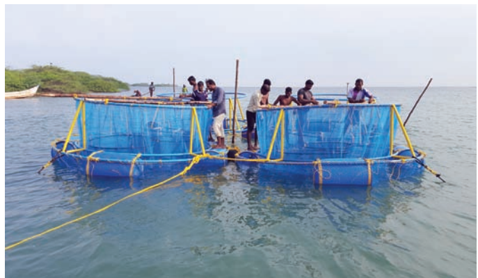
Installation of GI cage at site
