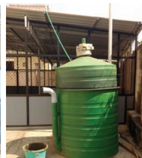
Biowaste management unit set up at Mangalore Research Centre
