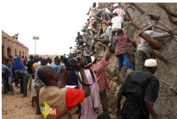
An ORTM photojournalist recording workmen applying earth plaster at the Tomb of Askia in Gao, Mali, 2014 © UNESCO/ B. Modibo
