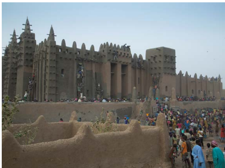
Earth plastering at the Great Mosque of Djenné, 2015 © UNESCO / B. Modibo
