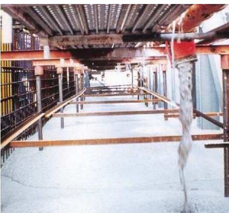
Highly workable concrete for anchorage body
