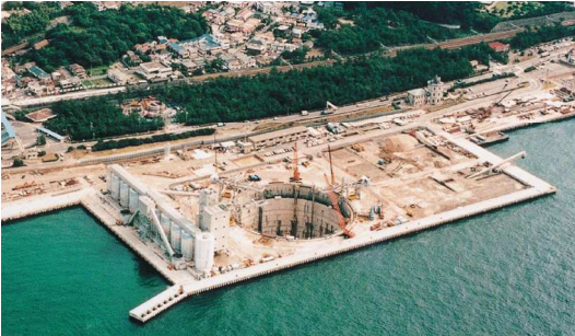
Distant view of 1A anchorage foundation work
