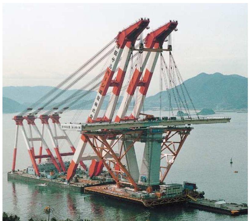
Large block erection of main girder connecting tower
