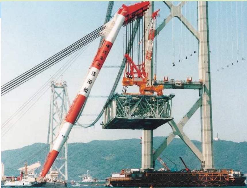
Large block erection near main tower
