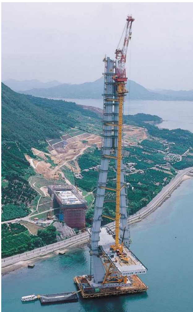
Completion of tower erection
