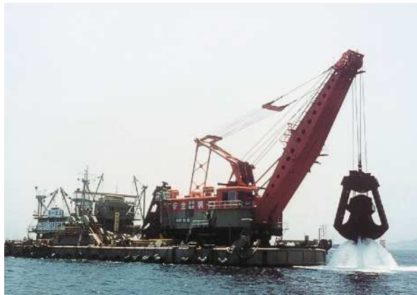
Excavation of the seabed using a large grab bucket dredger
