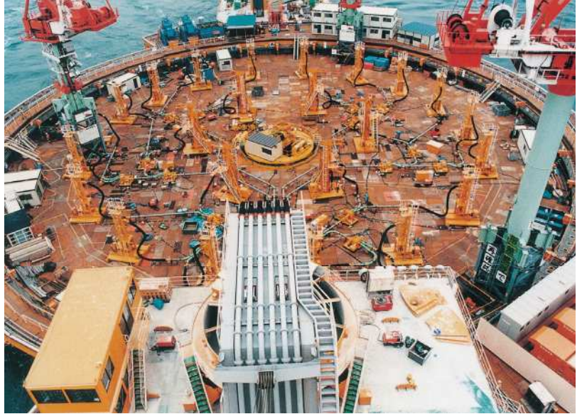
Casting underwater desegregate concrete
