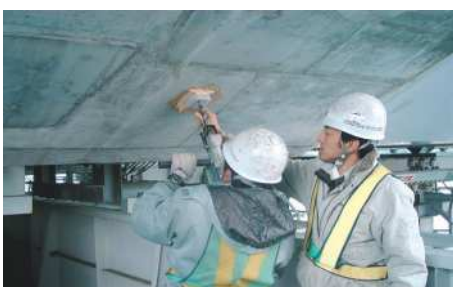
Measurement of chloride-ion
