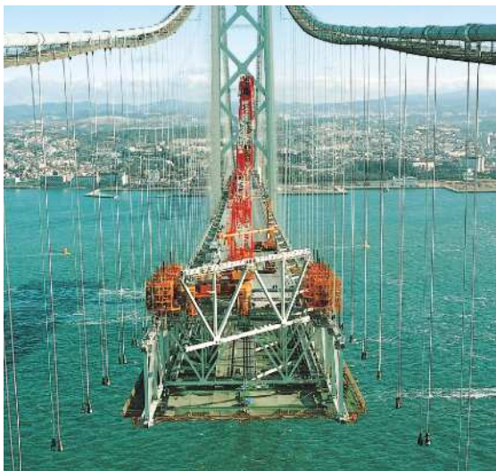
Plane element installation
