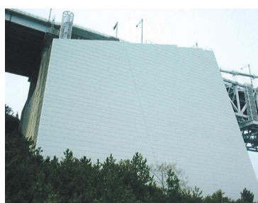
Paint coating on Ohnaruto 1A
