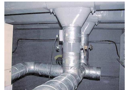
Air duct to U-rib
