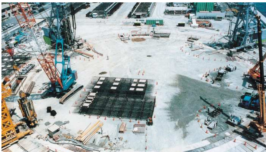
Excavation using underground slurry wall method
