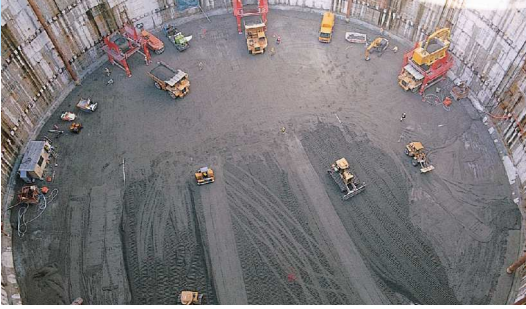
Inner concrete (Roller Compacted Concrete,RCC)
