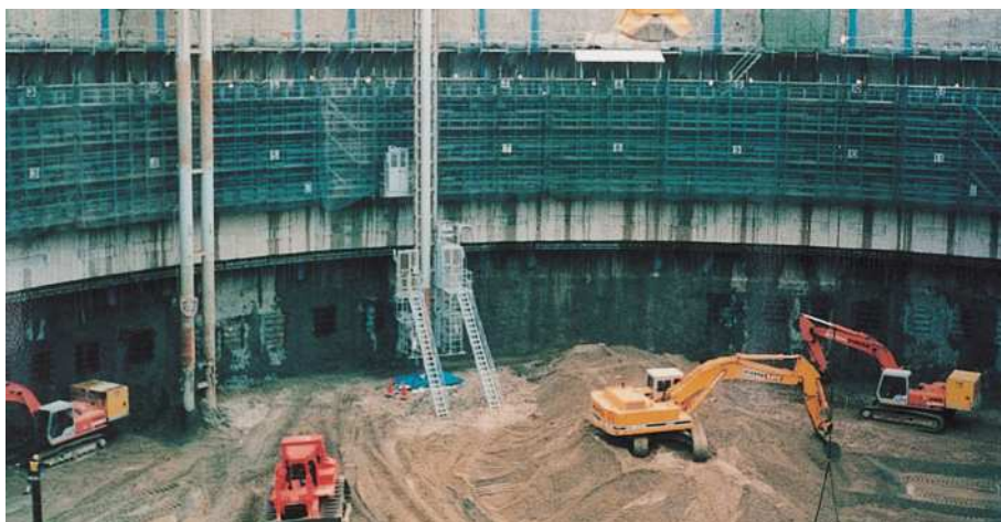
Excavation of inside of slurry wall
