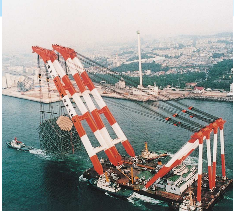
Transportation of cable anchor frame using a floating crane
