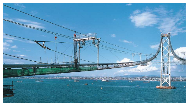
Erection of cable strand
