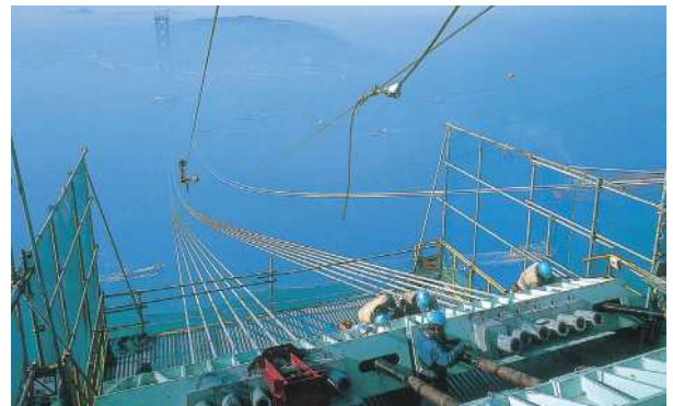
Completion of a catwalk rope
