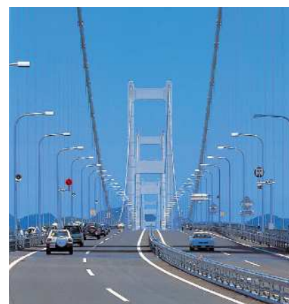
Kurushima Kaikyo Bridges (Nishi-Seto Expwy.)
