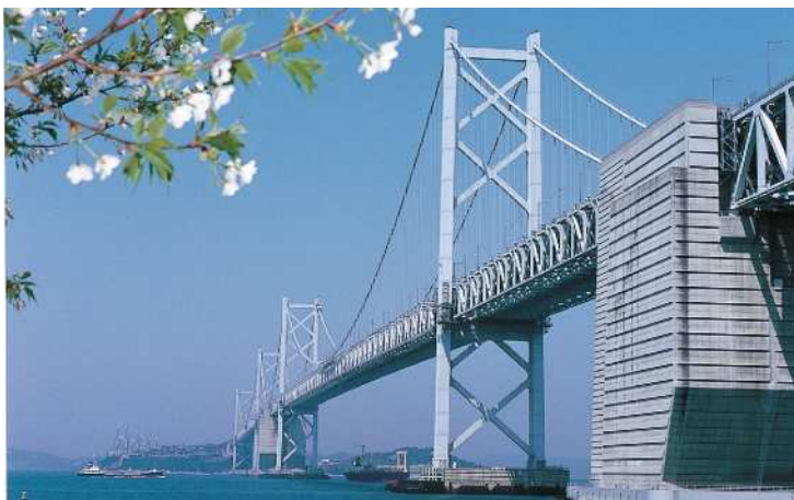
Kita & Minami Bisan-Seto Bridges
