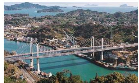
① Shin-Onomichi Bridge (completed in 1999, forefront) This is a steel cable-stayed bridge with a center span of 215m.
