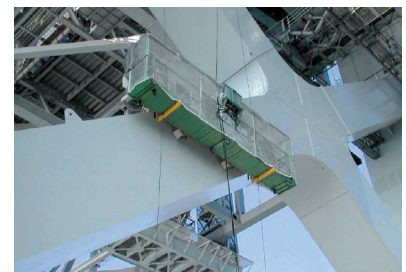
diagonal and horizontal member (work on sideboard of diagonal member)
