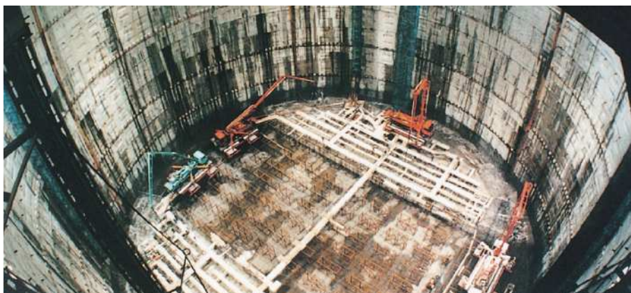
Construction of the bottom slab concrete
