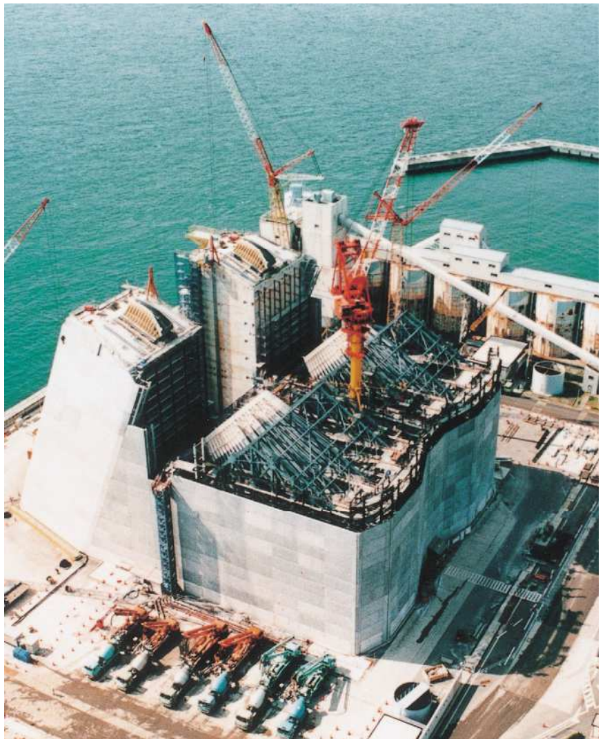
Distant view of 1A anchorage work
