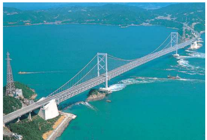
Ohnaruto Bridge (completed in 1985)
