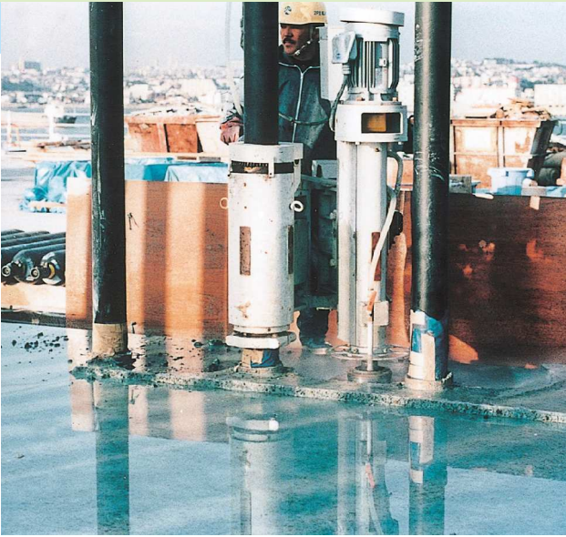
Grinding concrete surface before installation of bottom plate
