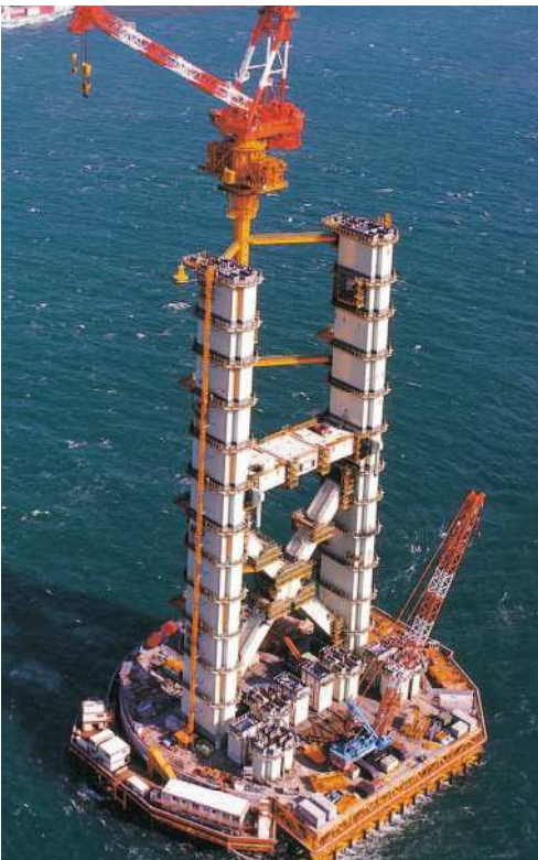
Climbing crane used for tower erection
