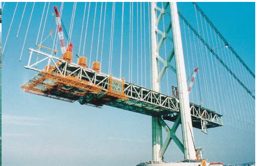
Transportation of plane element
