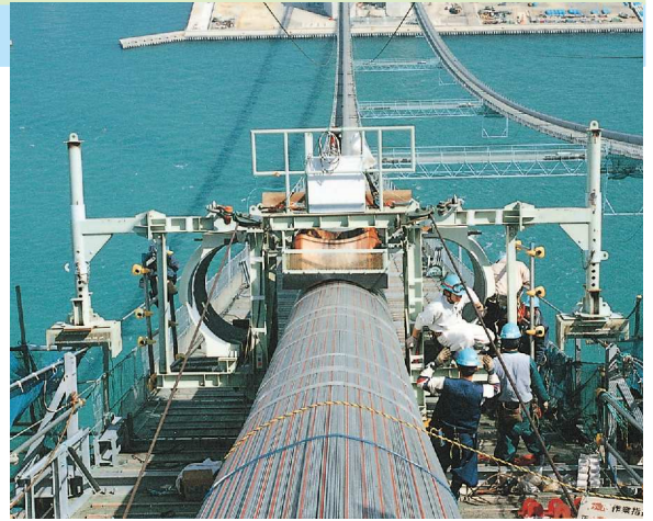
Installation of cable band
