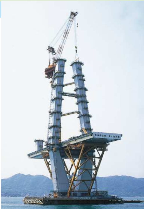
Erection of tower
