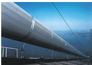
Main cable just constructed
