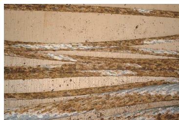
Corroded inner layer strands
