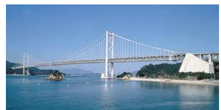
② Innoshima Bridge (completed in 1983) This is a 3-span, 2-hinged stiffening truss suspension bridge with a center span of 770m.
