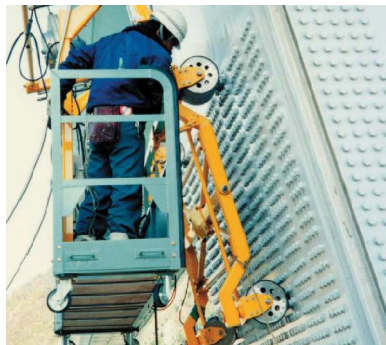
Gondola for tower wall
