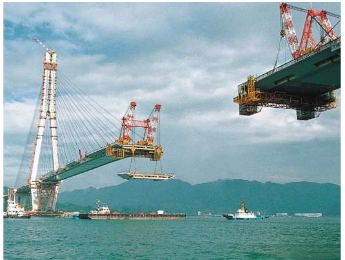
Balanced cantilever erection
