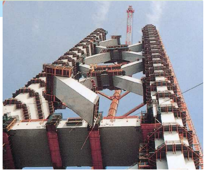
Erection of diagonals
