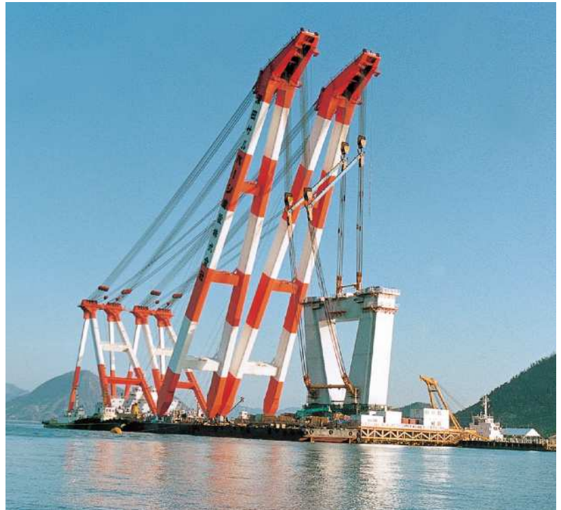
Large block erection of bottom part of tower
