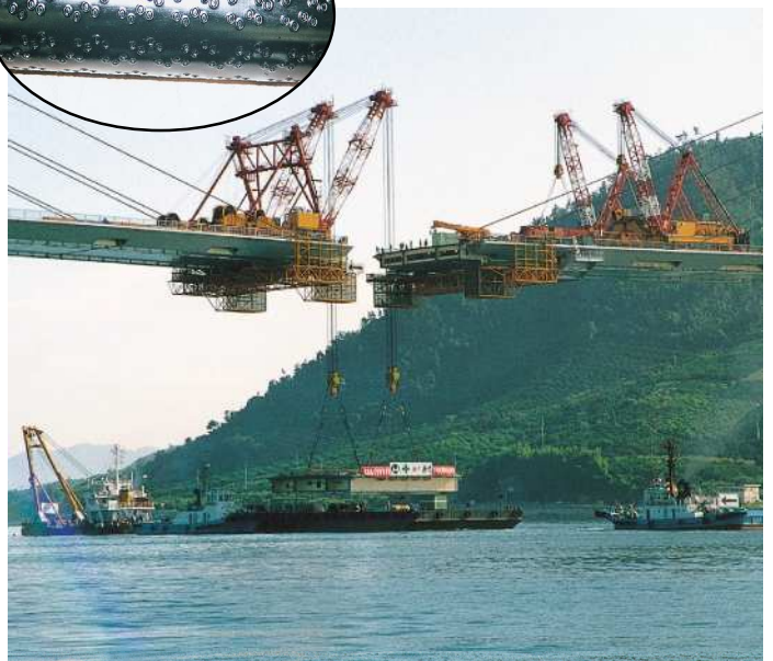
Erection of closure segment
