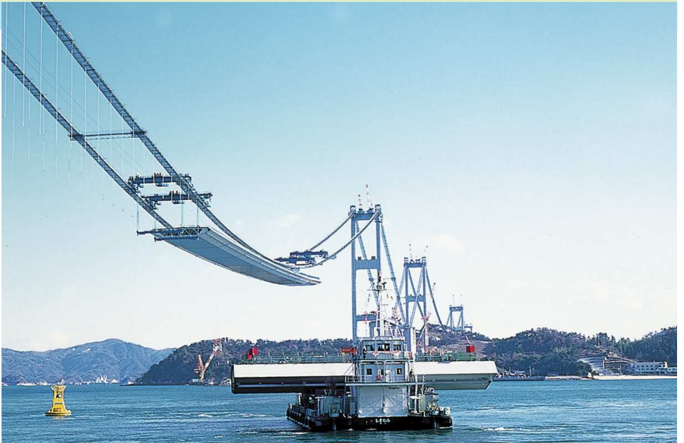
Start of hoisting up by lifting beams
