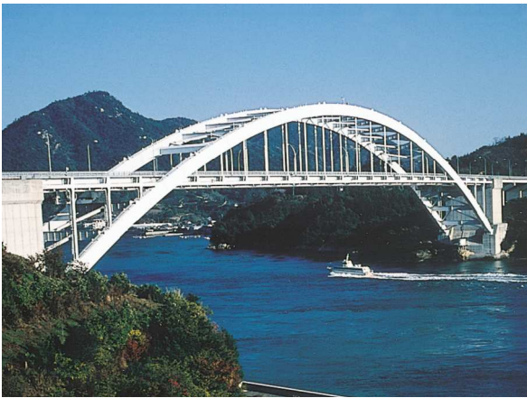
⑤ Ohmishima Bridge (completed in 1979) This is a steel, 2-hinged, solid-rib arch bridge with an arch span of 297m.
