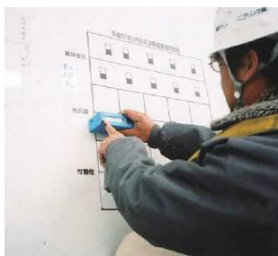
Site survey for painting
