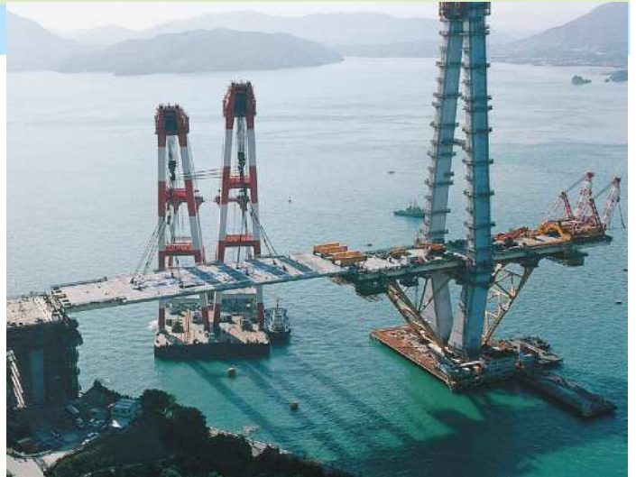
Large block erection of side-span girder
