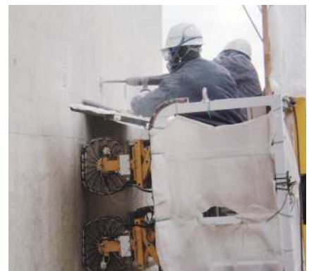
Under repair work
