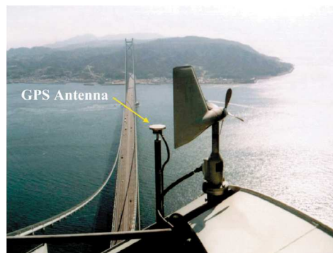
GPS sensor on Akashi-Kaikyo Bridge
