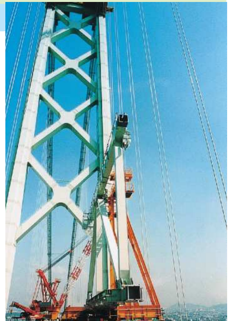
Transportation of plane element
