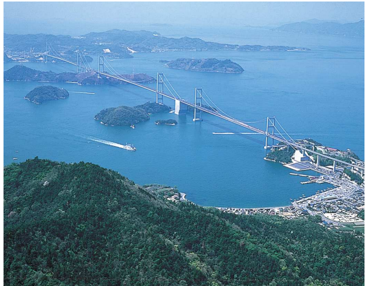
⑦ Kurushima Kaikyo Bridges (completed in 1999) The Kurushima Kaikyo Bridges consist of three suspension bridges, they are structurally connected by a couple of double anchorages.
