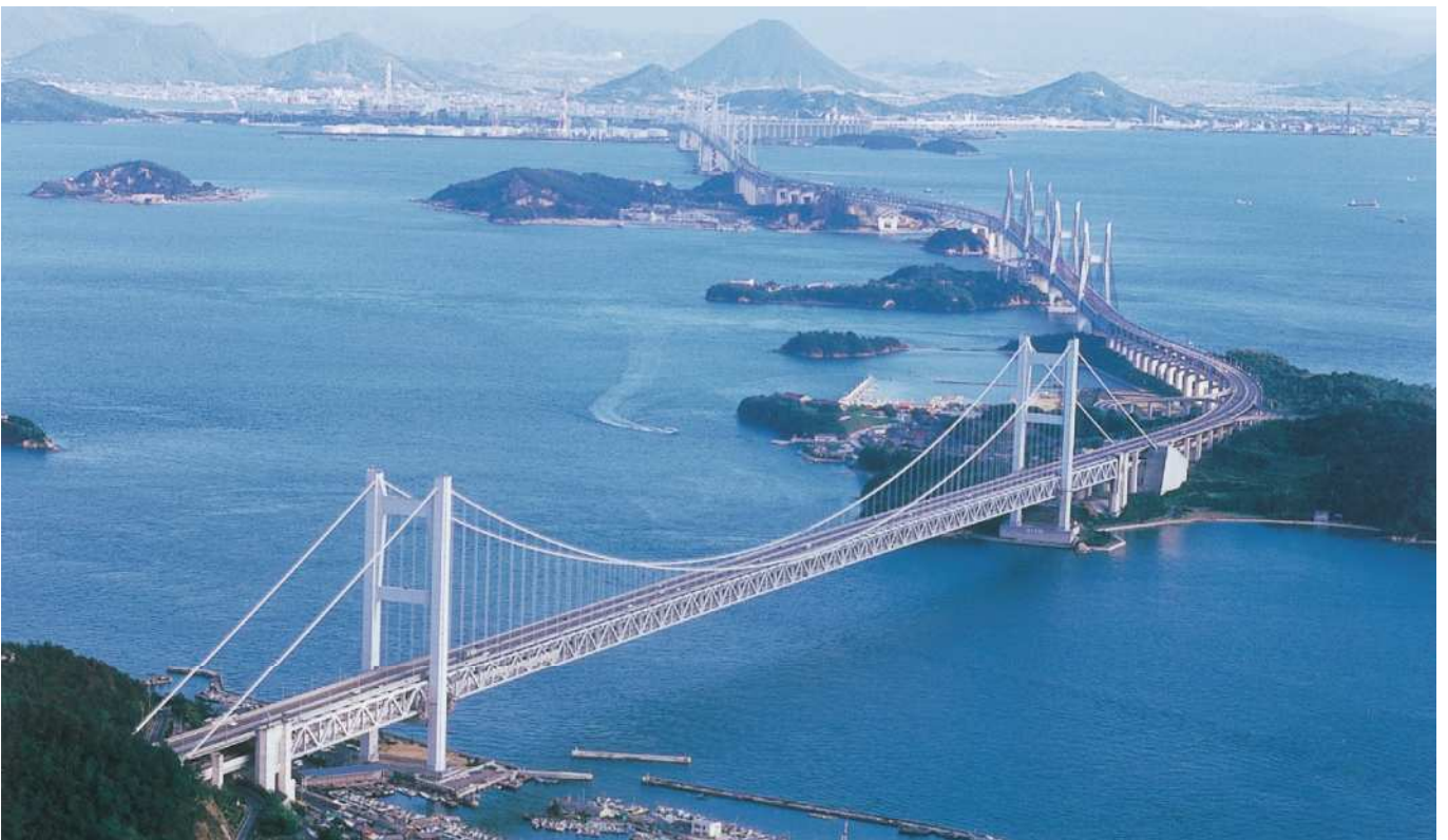
Panoramic View of the Seto-Ohashi Bridges (from Honshu-side, completed in 1988)
