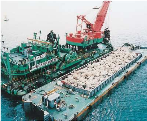
Dropping rip-rap (scour protection)
