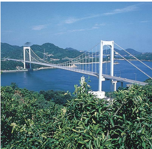
⑥ Hakata-Ohshima Bridge (completed in 1988) This is a single span box girder suspension bridge with a center span of 560m.
