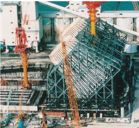
Concrete casting of anchorage body
