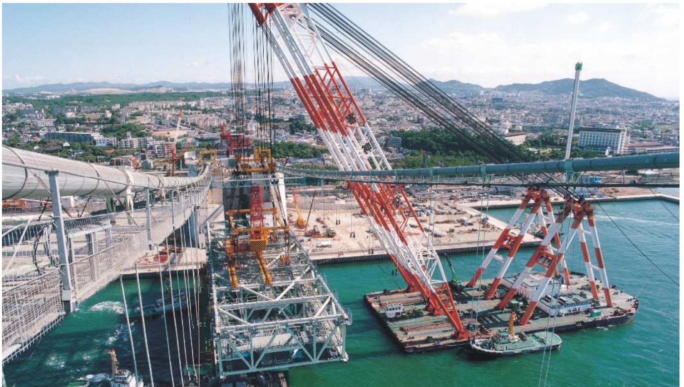
Large block erection near 1A anchorage
