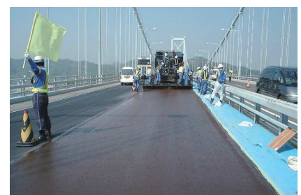
Micro-surfacing method
