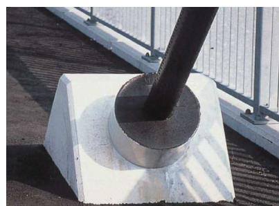
Vibration control by high-damping rubber
