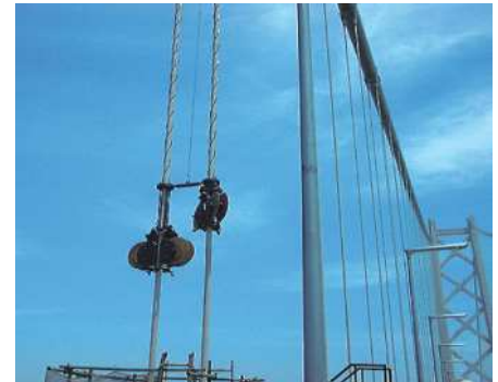
Installation of trip wire
