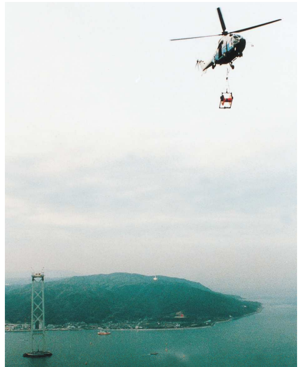
Spanning of a pilot rope across the strait by a helicopter
