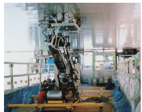
Painting robot for box girder
