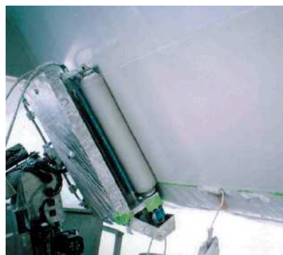
Painting work on inclined web
