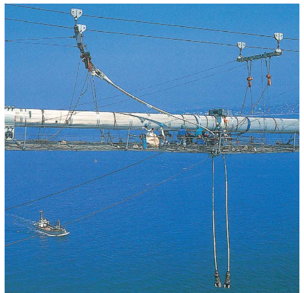
Installation of hanger rope
