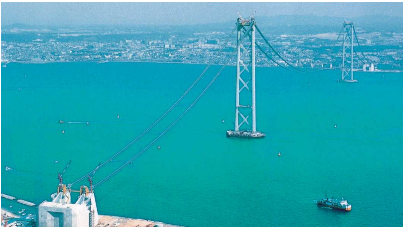
Distant view of cable works
