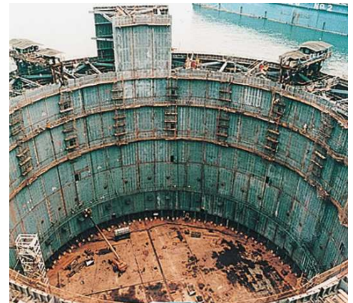
Manufacturing a steel caisson
