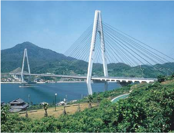
③ Ikuchi Bridge (completed in 1991) This is a composite girder cable-stayed bridge, center span of steel and side spans of concrete.
