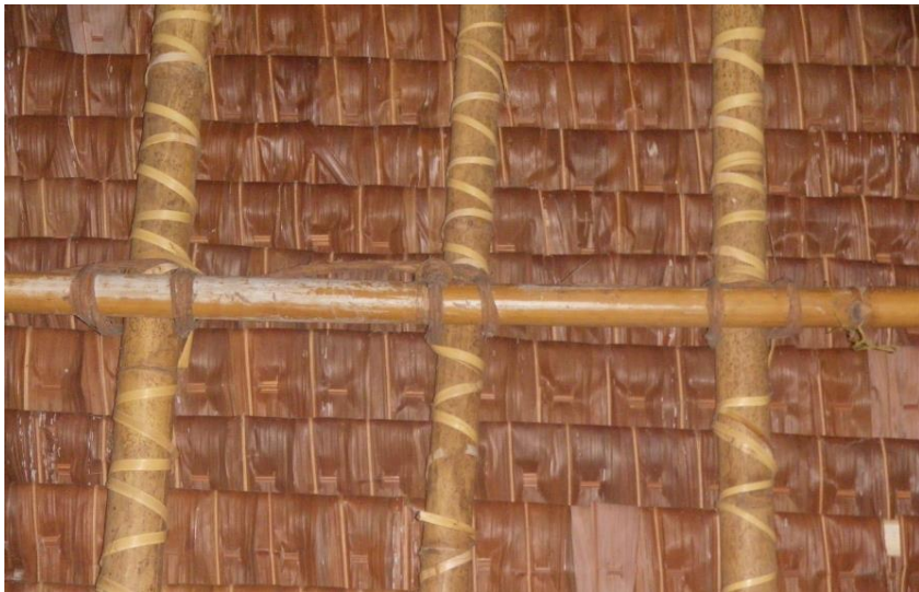
Figure 7: Layers of thatch panels are mich 'tied' to bamboo trusses inside a home
