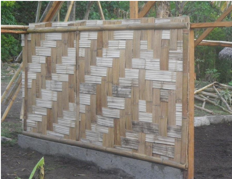
Figure 6: A ner (EB) 'wall' panel installed on a new home
