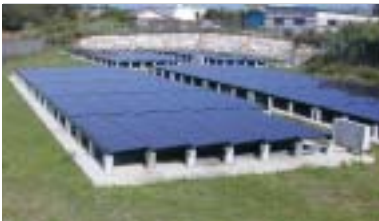
Field tests on an industrial solar power system are being carried out at a facility on Kita-Daito Island.
