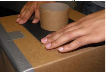
Hot glue the lens barrel collar over the hole using the lens barrel to help align it.
