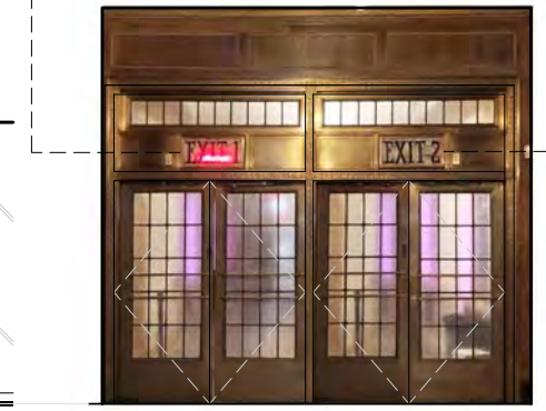
③ WEST ELEVATION RETAIN EXISTING DOORS
