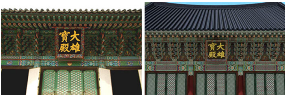
Figure 32: A photograph of bracket system of the main Buddha hall (left) and my graphic work image (right).
