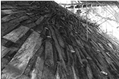
26) Planking for roof foundation Small piece of woods put on top of the roof to give a slope to a roof.
