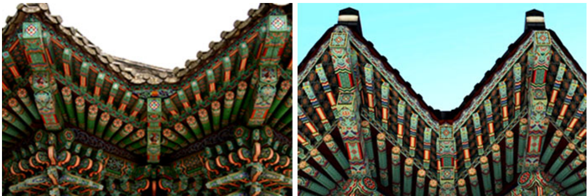
Figure 33: A photograph of double eaves and rafters of the main Buddha hall (left) and my graphic work image (right)
