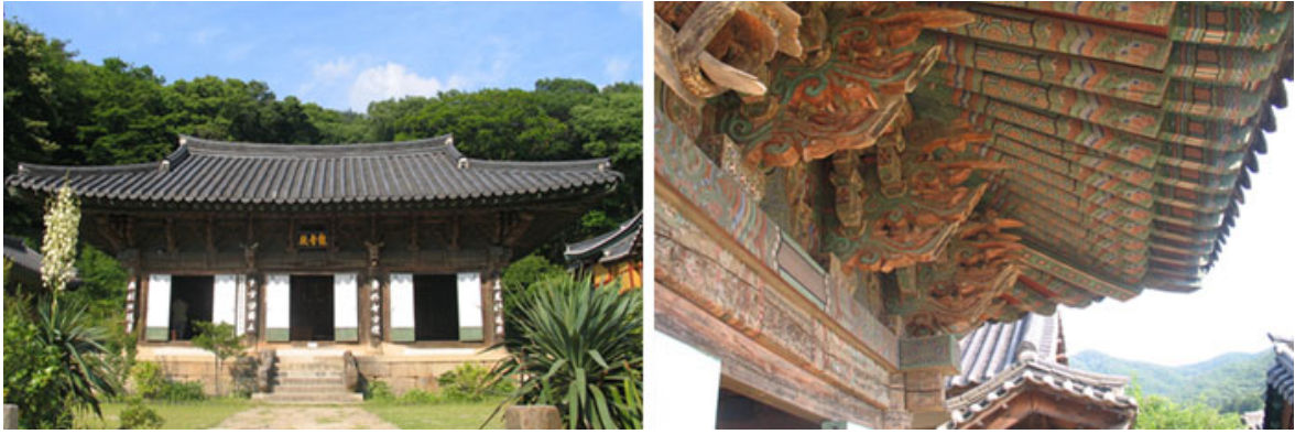
Figure 65: Gwanumjern and its bracket systems
