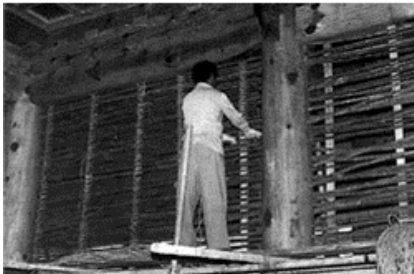
28) Plasterwork for walls.
