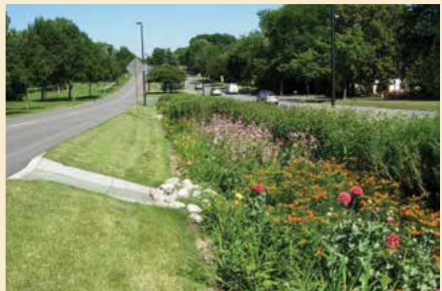
Example of a bioswale to increase water absorption in a highway median. Photo Credit: Aaron Volkening used under CC BY 2.0.
