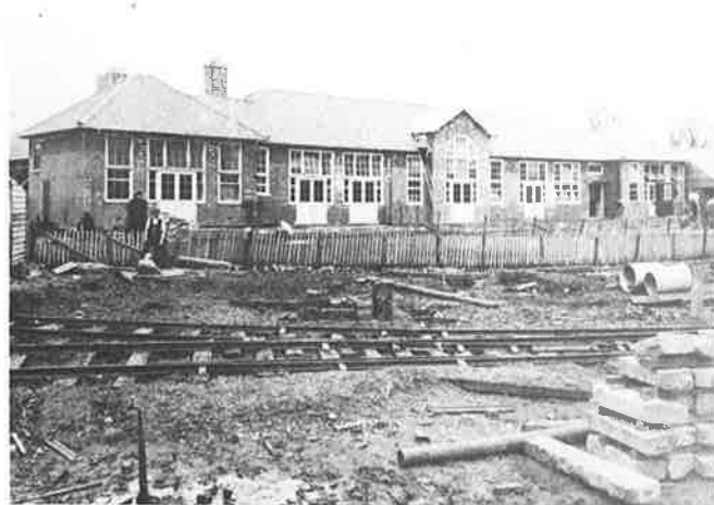
Rangefield School, Downham, under construction
