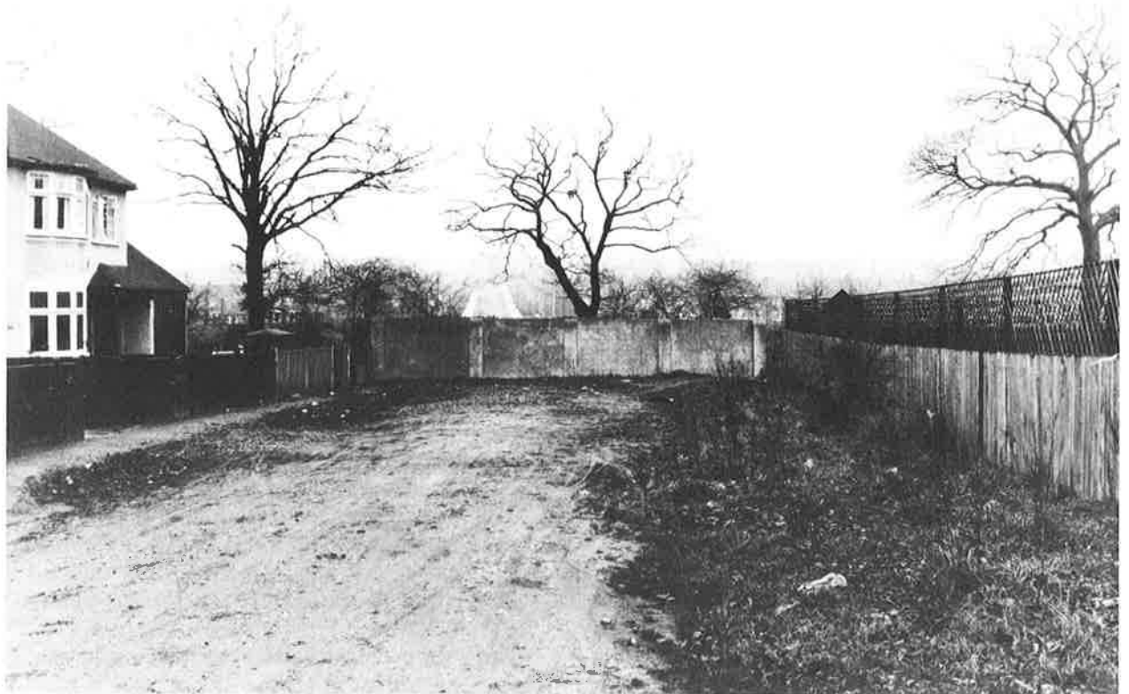
The 'Downham Wall' built by private residents to distance themselves from council tenants. General view from Alexandra Crescent, Bromley, 1927
