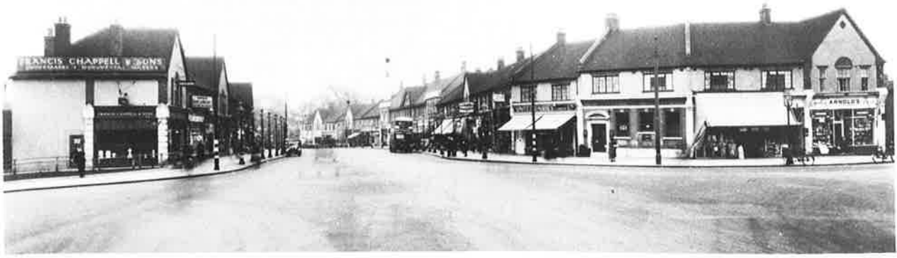
Shopping Centre, Bromley Road, Downham, 1930
