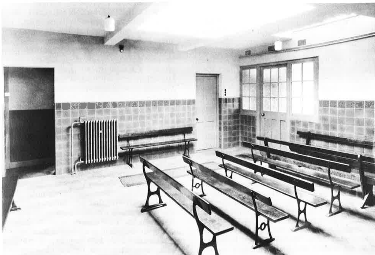
Downham Health Centre. Interior of Female Waiting Room, 1932
