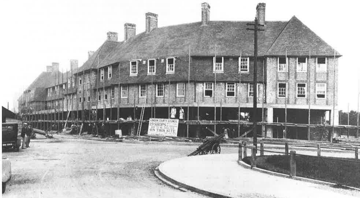
Shops being erected at Green Lane North, St Helier 1931
