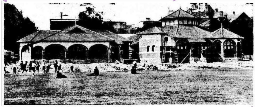
The octagonal refreshment kiosk and dressing rooms (five for men and one for women) facing the Esplanade, close to Barrack-street. The contract price was £5,991. Tenders are being called for the leasing of the premises, which the council is confident will return more than interest on the expenditure, notwithstanding adverse criticism. The architect was Mr. L. B. Cumpston.
