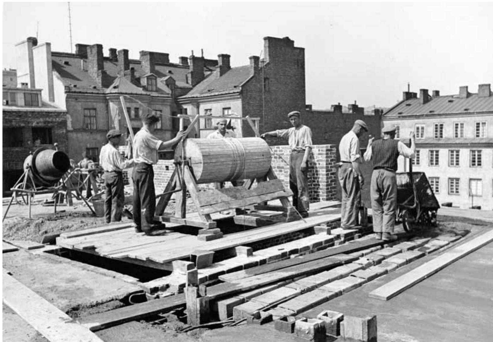
Budowa domu - roboty betonowe Building a house - working with concrete.
