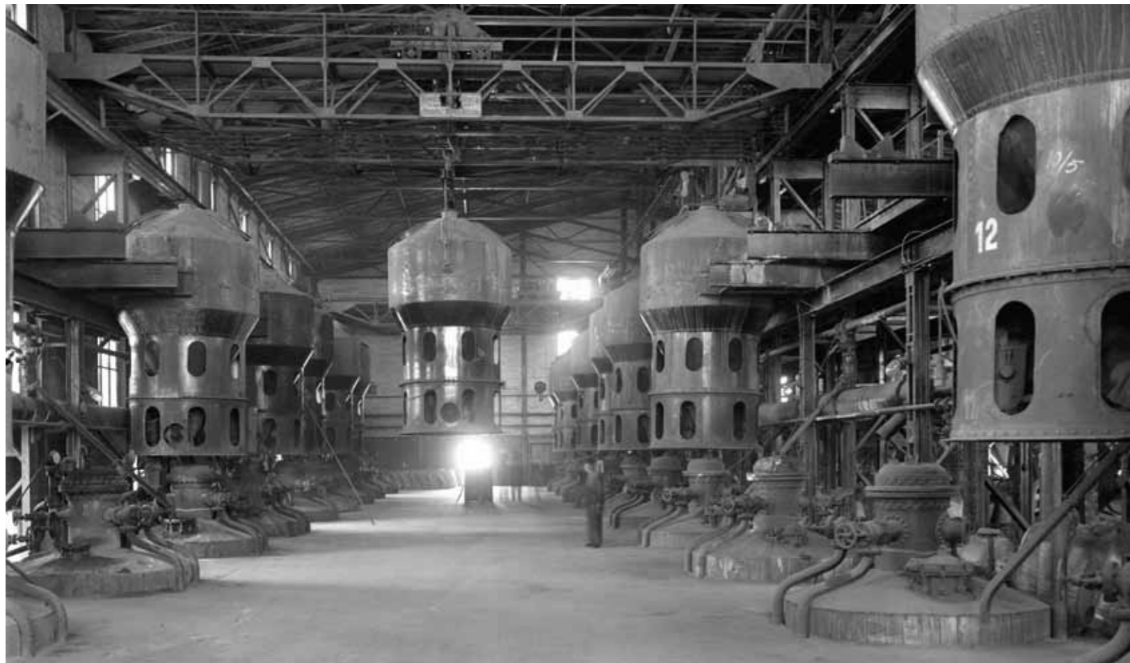
Amoniakarnia, Chorzów Ammonia stripping facility, Chorzów.
