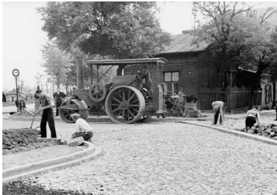
Roboty brukarskie, Warszawa Setting cobblestone, Warsaw.
