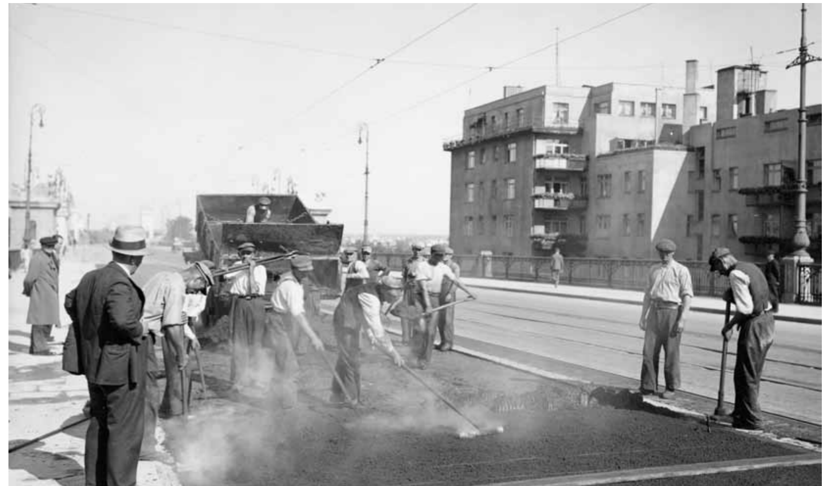
Roboty asfaltowe, Warszawa Asphalt work in process, Warsaw.
