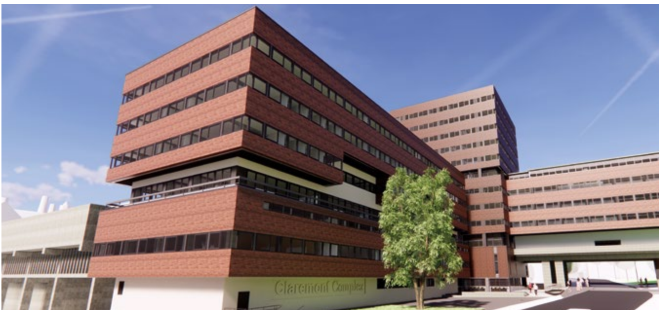
Phase 1 of the Claremont–Daysh refurbishment is due for completion in 2020.
