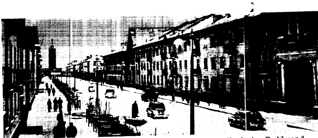
Figure 4. The town of Inta on the Kotlas-Vorkuta Railroad.
