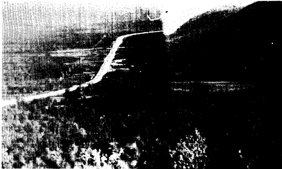
Figure 68. A distant view of the Murmansk-Pechenga railroad at a point east of the Pechenga River. (1955)
