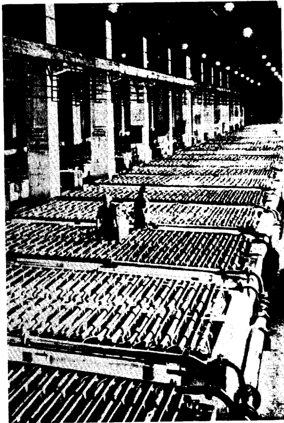
Figure 27. Interior of the electrolytic refinery of the Noril'sk nickel combine. (1956)
