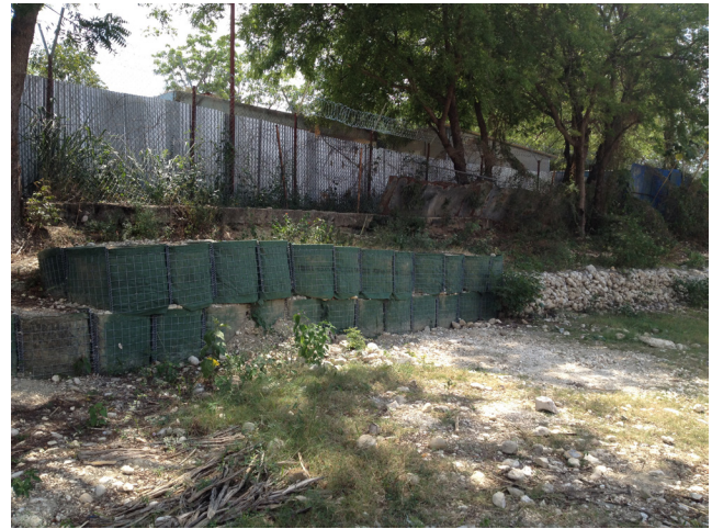
Barricades along the perimeter of the MINUSTAH camp.
