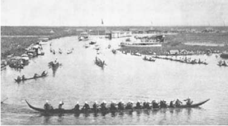
Opening the delta: works of canalization, c. 1900.
