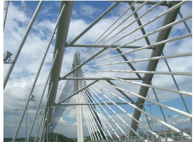
Figure 1: Stays crossing bracing members
