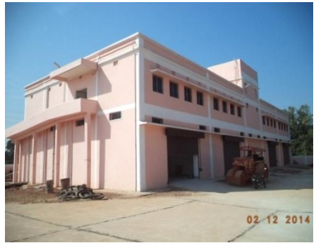
Jatani Godown-cum-MCS in Jatani Block under NCRMP, World Bank funded.
