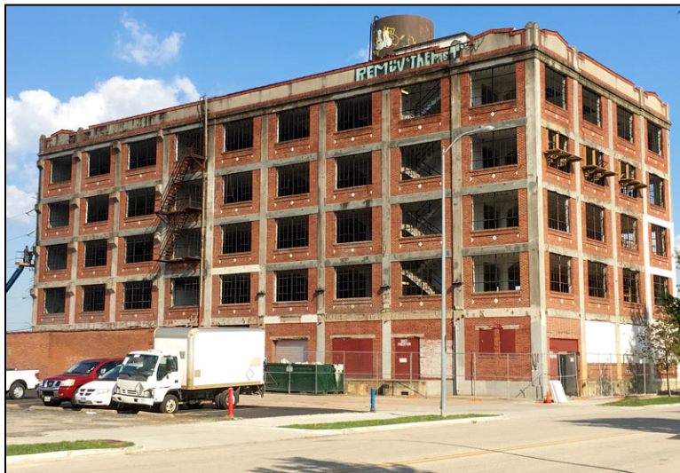
Figure 6-11 Cheek Neal Coffee Company historic building in redevelopment
