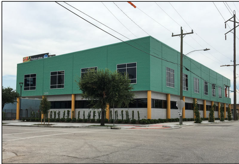
Figure 6-10 SEARCH facility under construction in 2017
