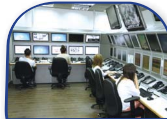
Control Center/ Dispatch Services
