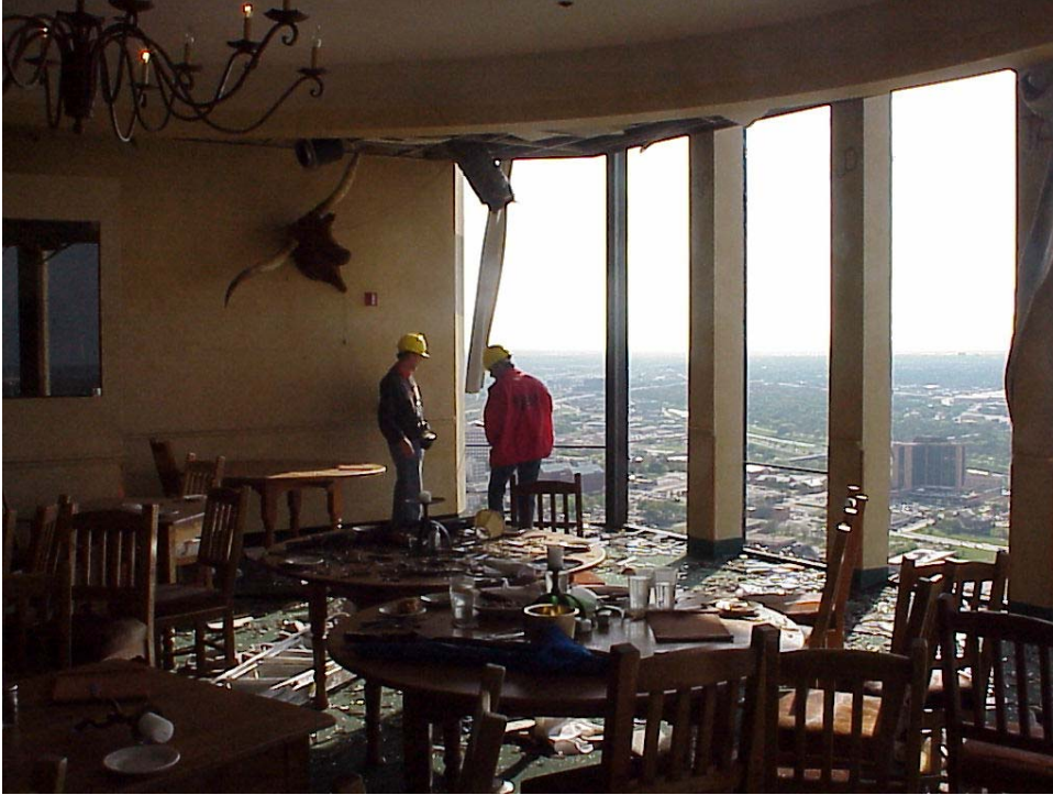
Figure A27. Inside top floor restaurant of Bank One looking southwest.
