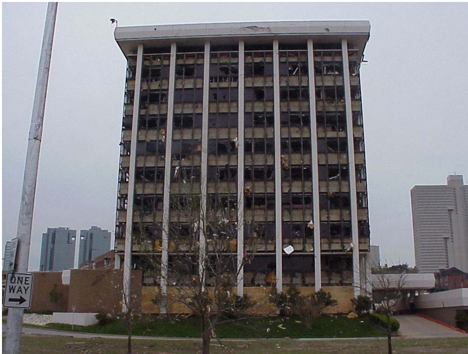
Figure A18. West face of Mallick Tower.
