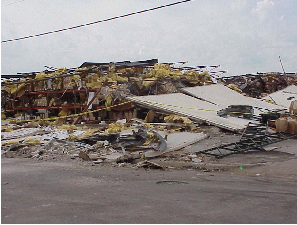
Figure A3. Northeast corner of Sweet Shop Factory.
