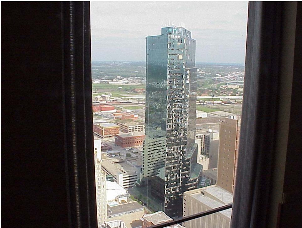
Figure A28. Southwest face of UPR Tower from Bank One
