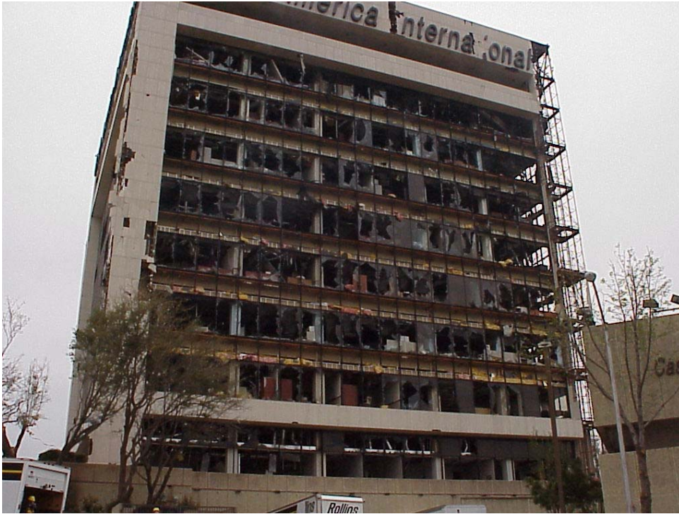
Figure A5. Northwest face of Cash America International building.
