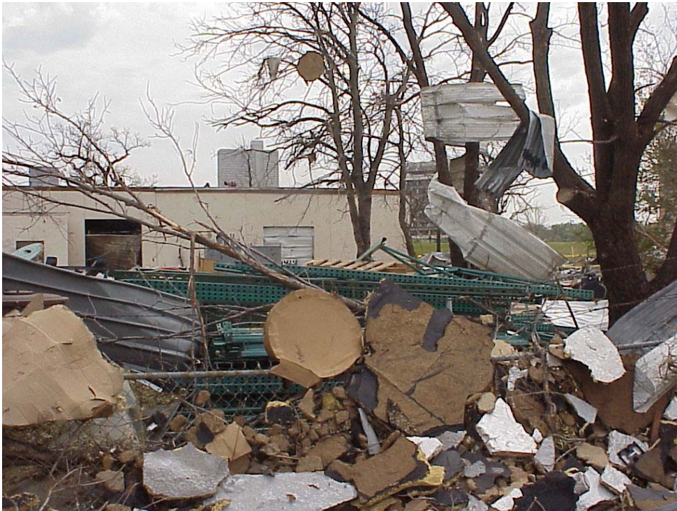
Figure A4. Debris from Johns Manville warehouse in Harrold Street.
