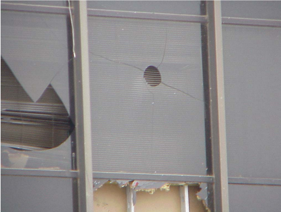
Figure A19. Debris impact Point in vision glass on Mallick Tower.
