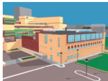
Fig 3 Artist's impression of final Conservation Studios showing the zigzag windows providing north light to the upper Conservation Studios. Sound Studios on the lower floor are built using blockwork, thermal and acoustic insulation and sit on reinforced concrete slabs floating on acoustically isolating rubber pads some 600mm thick. Image reproduced with kind permission of the British Library Board.
