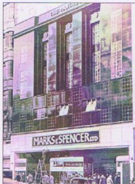
The shop opened in 1938 but suffered extensive interior wartime damage
