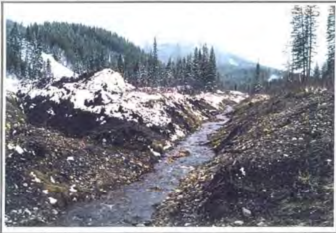
Photo 9 Channelized portion of Little Hopeful Creek (Reach 2) May 8, 1996.
