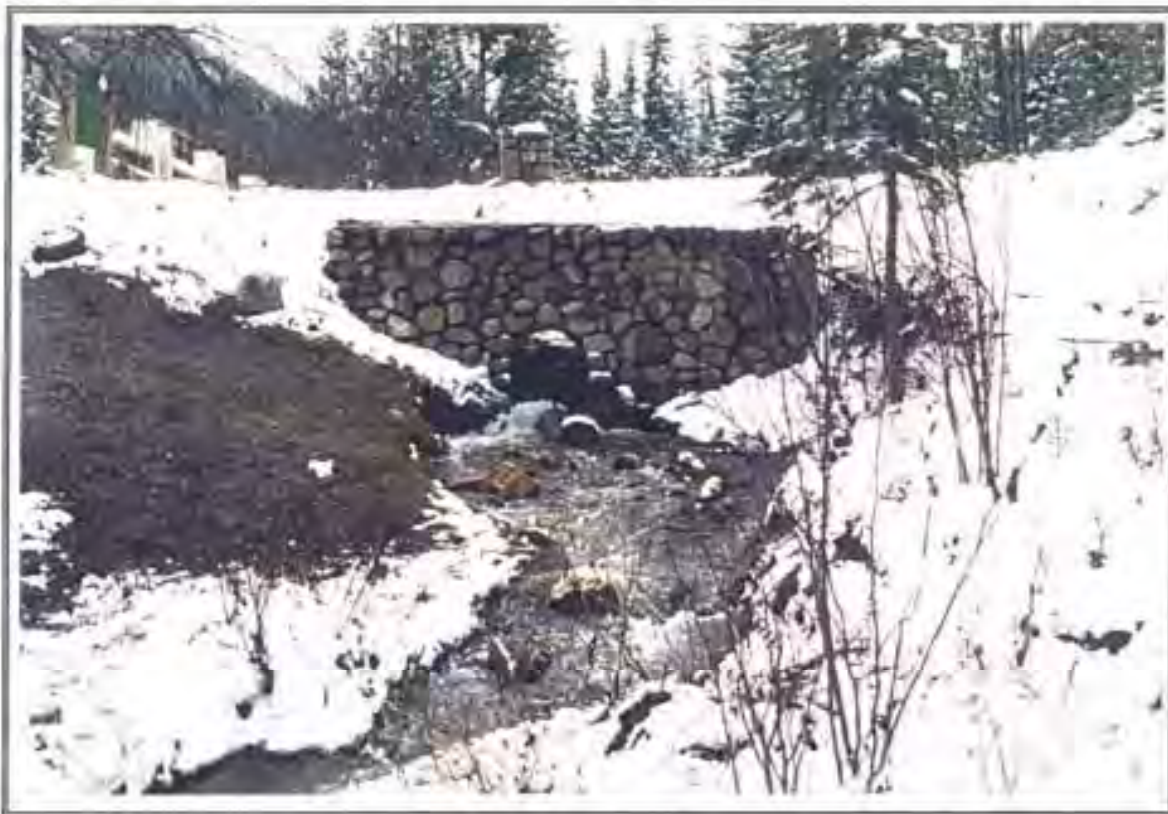
Photo 6 Culvert near mouth of Little Hopeful Creek (Reach 1) May 8, 1996.
