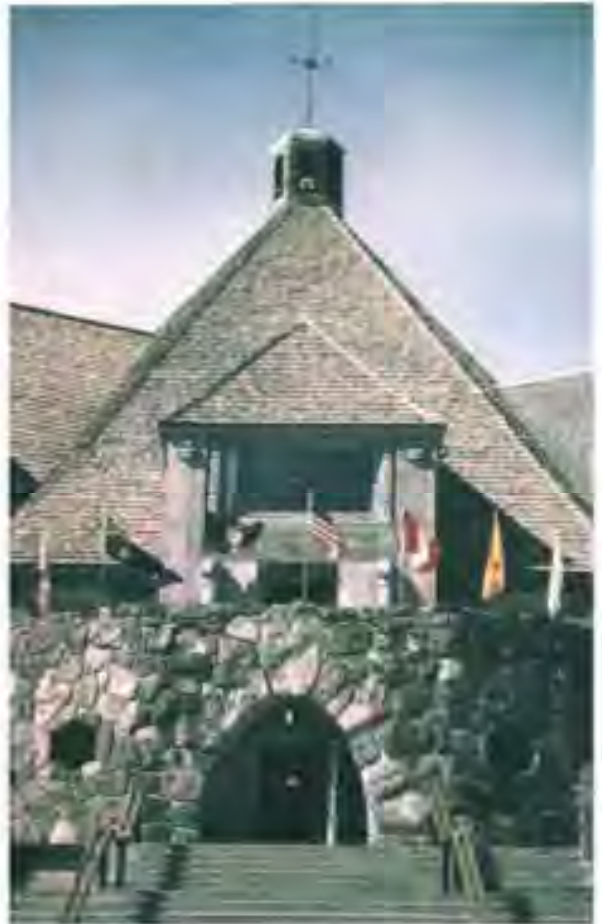
MOUNT HOOD'S TIMBERLINE LODGE PROVIDES ARCHITECTURAL INSPIRATION FOR THE FUTURE CONFERENCE CENTRE HOTEL.
