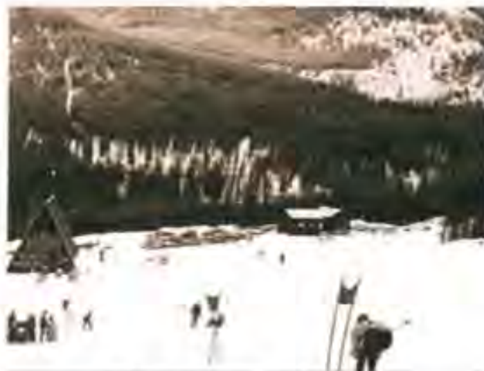
VIEW OF ORIGINAL DAY LODGE
