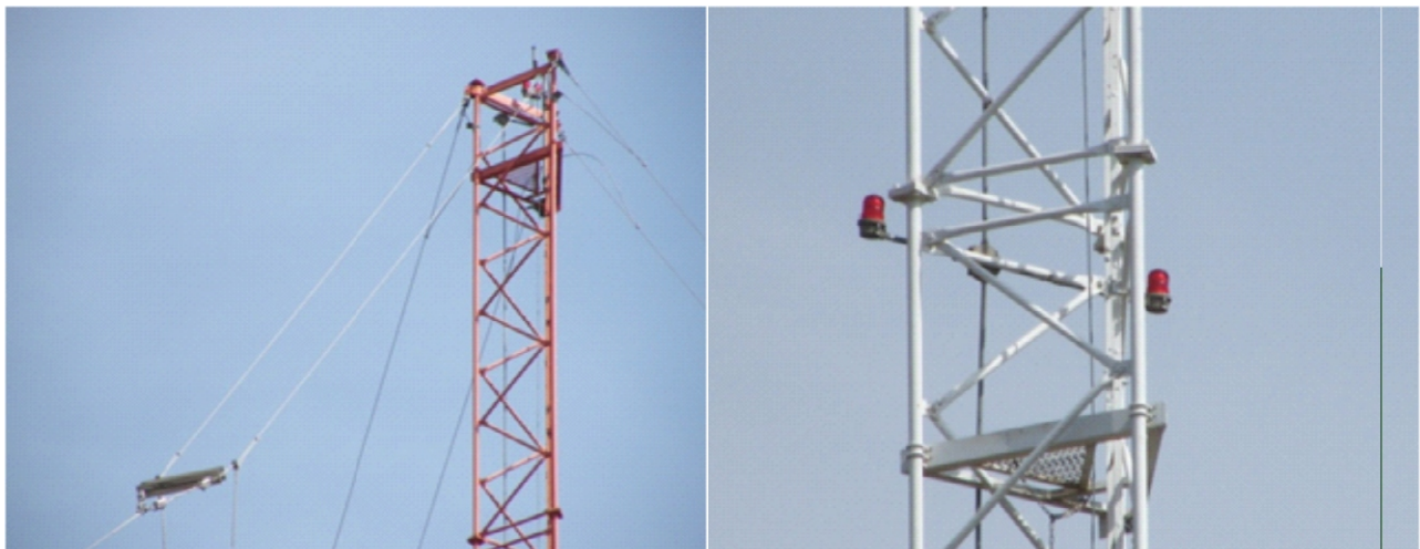
Figure 28: Top part of the mast painted red and lighted part of the mast painted white showing lights
