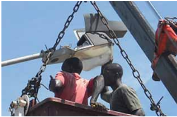
BB Electricians Changing The Lamps
