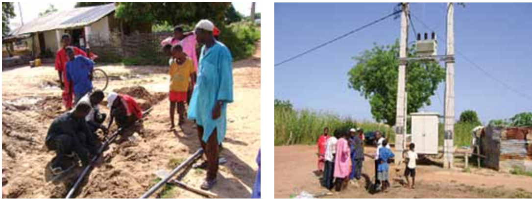
FIGURE 17 Fatoto community replacing faulty water distribution pipe through community work
