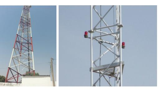
Figure 19: Tower showing alternate red / white aviation safety paint
