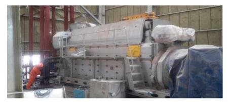
Figure 22: The new MAN 2.3MW engine HFO engine at Farafenni being installed
