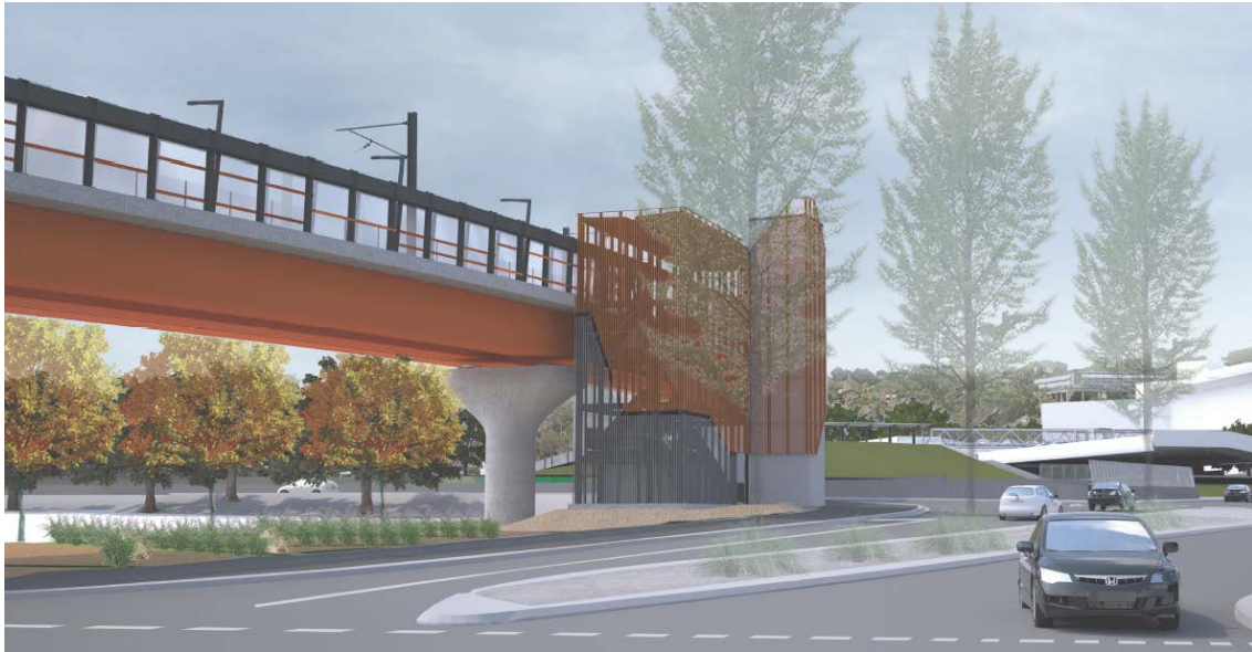
Figure 5: Viaduct and stair/lift core (Laffers Triangle)
