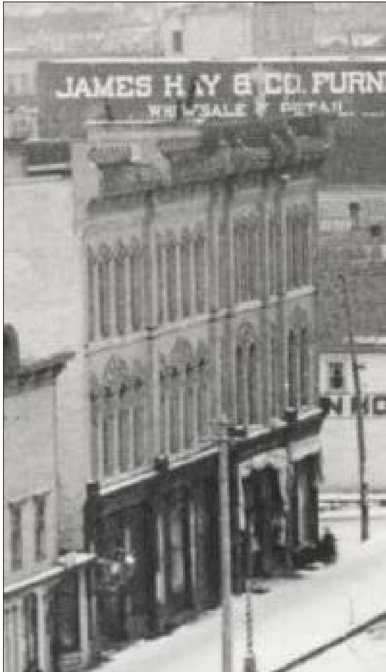
Plate 8 – Fortune Block, 232 Main Street (right) in 1892 still featuring the original retail layout on the east façade. ( Archives of Manitoba, Victor Acker Collection- 2, N842. )
