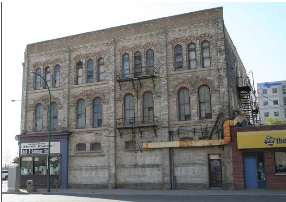
Plate 15 – Fortune Block, 232 Main Street, north façade, 2015. (M. Peterson, 2015.)
