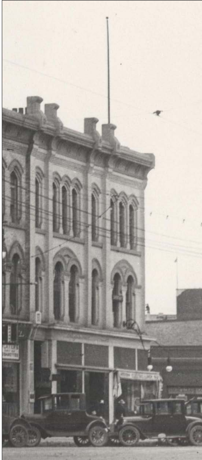
Plate 9 – Fortune Block, 232 Main Street, 1926. Elements of the cornice have been removed. (Courtesy of the Archives of Manitoba, Thomas Burns Collection- 542.)
