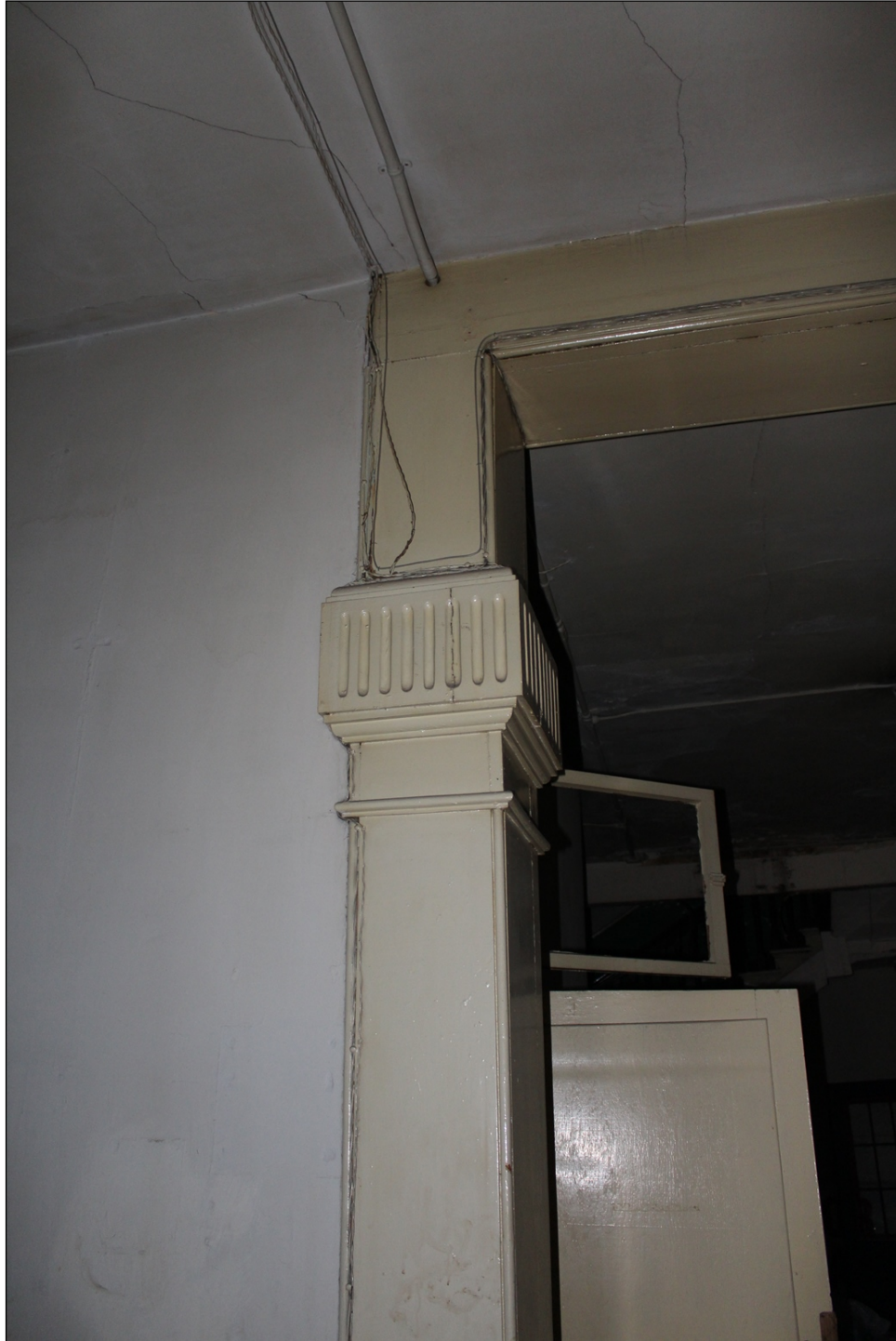
Plate 23 – Fortune Block, 232 Main Street, detail of second floor hallway, 2015. ( M. Peterson, 2015. )
