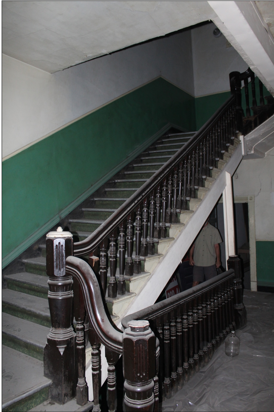
Plate 19 – Fortune Block, 232 Main Street, second floor staircase, 2015. ( M. Peterson, 2015. )
