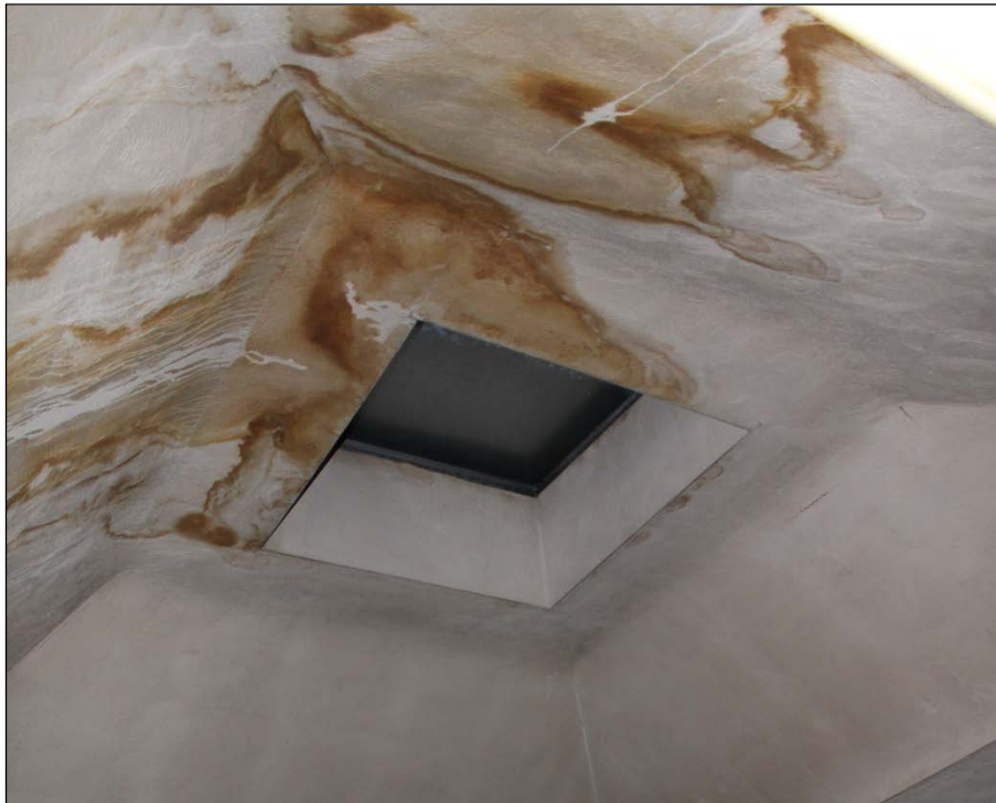
Plate 21 – Fortune Block, 232 Main Street, third floor skylight (now closed), 2015. ( M. Peterson, 2015. )
