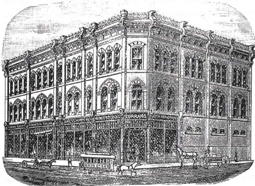
Plate 7 – An 1884 drawing of the Macdonald and Fortune Blocks, Main Street. Note the familiar retail front of the ground floor with its large display windows. The entrances do not appear to be recessed. ( Archives of Manitoba. )
