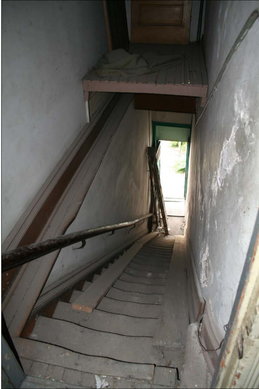
Plate 22 – Fortune Block, 232 Main Street, rear staircase, 2006. (M. Peterson, 2006.)
