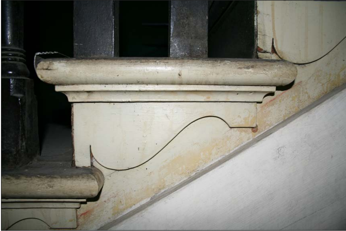
Plate 20 – Fortune Block, 232 Main Street, detail of second floor staircase, 2006. ( M. Peterson, 2006. )
