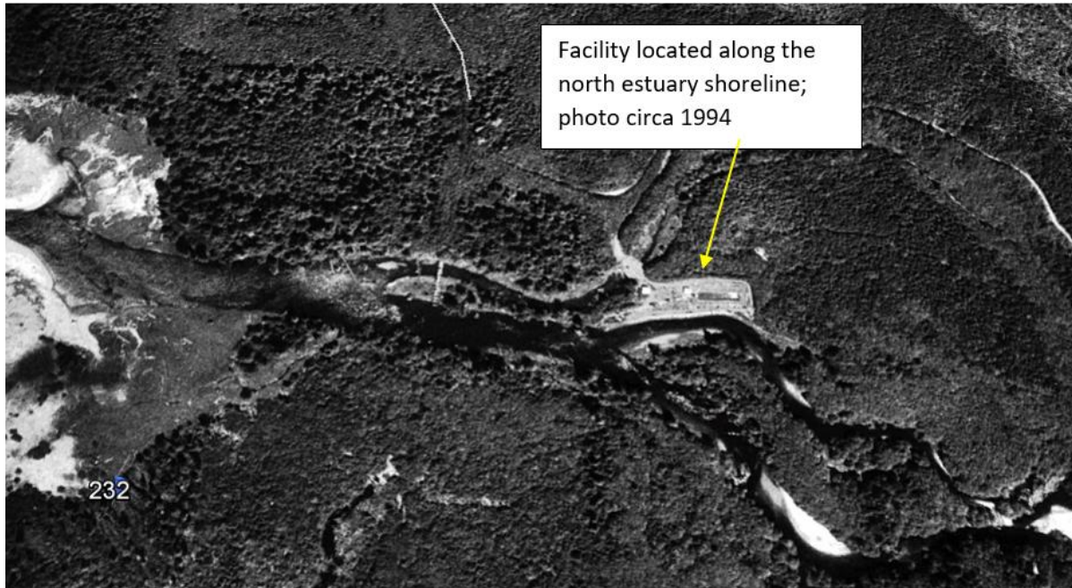
Figure 37. Facility along the north shore of R1, circa 1994.
