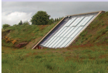
Figure 6 Set into the ridge, the house is surrounded by 350 million-year-old sandstone
