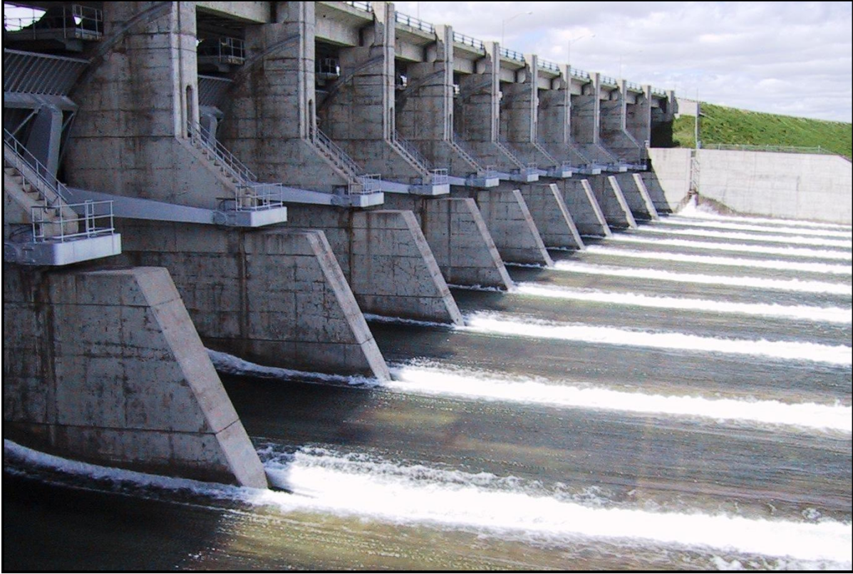
Figure 9 – Gardiner Dam Spillway
