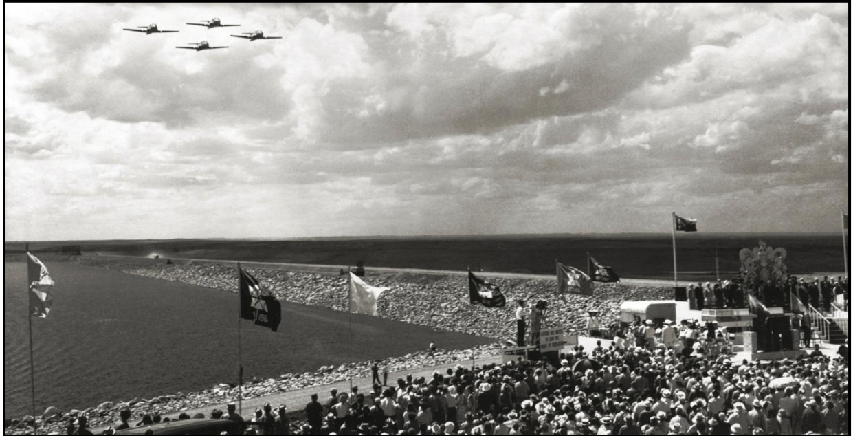
Figure 1: Gardiner Dam - Opening Ceremony July 21, 1967
