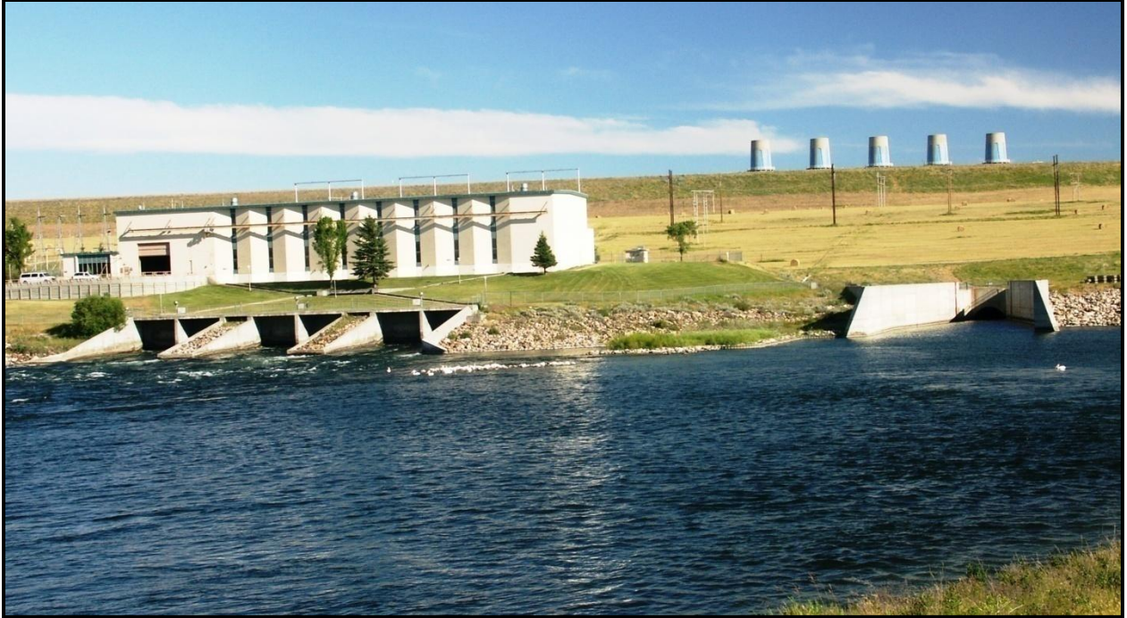
Figure 3 - Downstream View of Gardiner Dam SaskPower Coteau Structure
