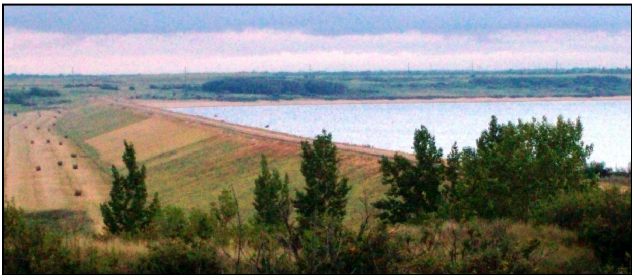
Figure 5 - South View Overlooking Qu'Appelle Dam
